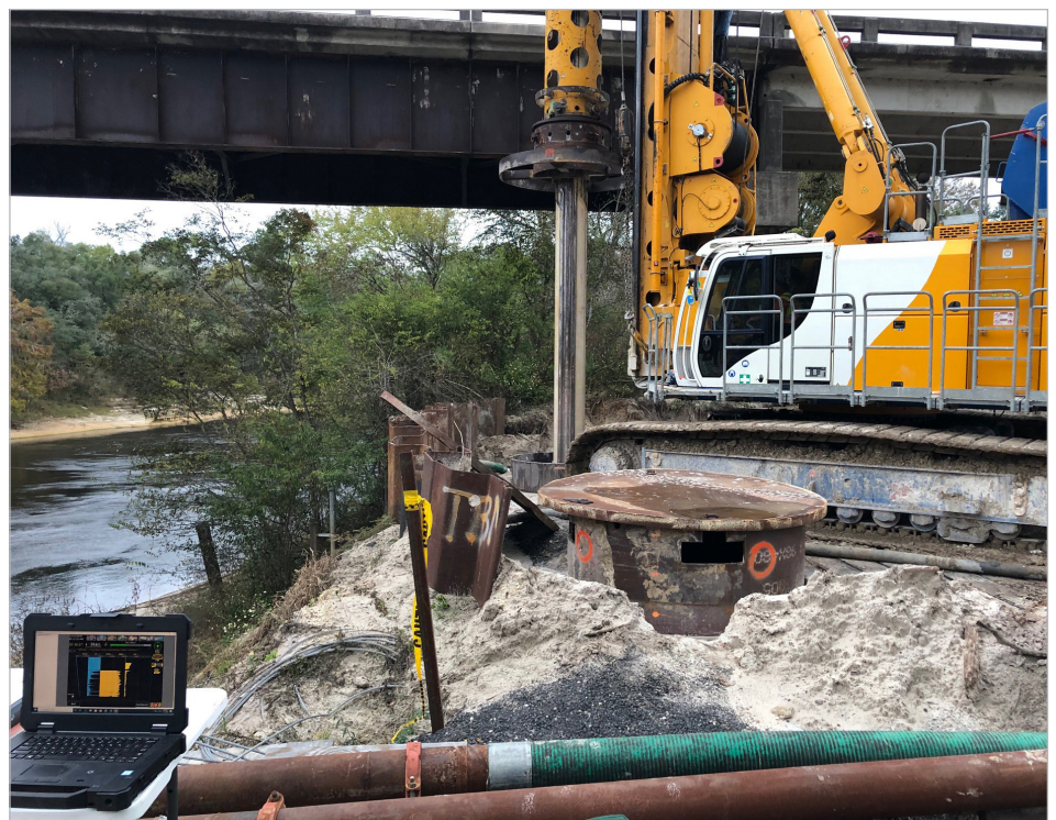
Florida DOT geotechnical engineers use measurement while drilling to gain more accurate and precise subsurface readings.
