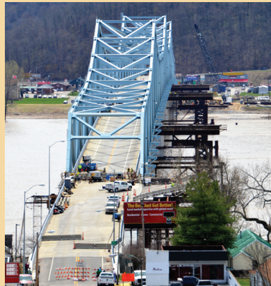
The Milton–Madison Bridge over the Ohio River is the longest in North America to be moved into place by sliding laterally, an ABC technique. The joint Indiana–Kentucky DOT effort also used design–build project delivery.
