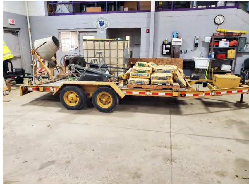
Outfitted trailer ready for catch basin repair project - Violet Township, Pickerington, Ohio
