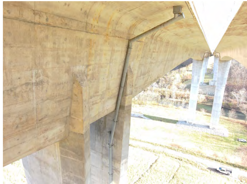
Drone Bridge Inspection of the Jeremiah Morrow Bridge, Warren County, Ohio - Ohio Department of Transportation
