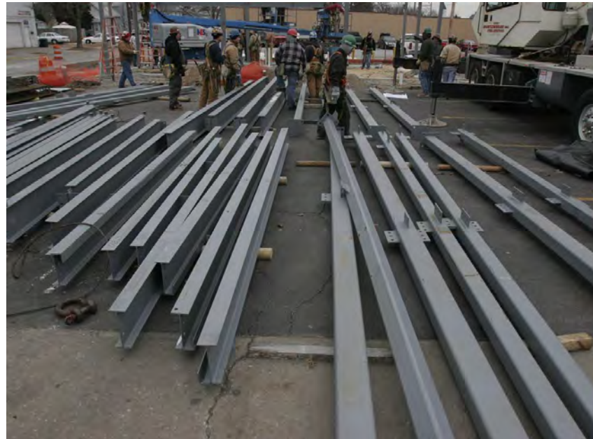
Upcycled bridge beams ready for a local construction project. - The Toledo Blade newspaper
