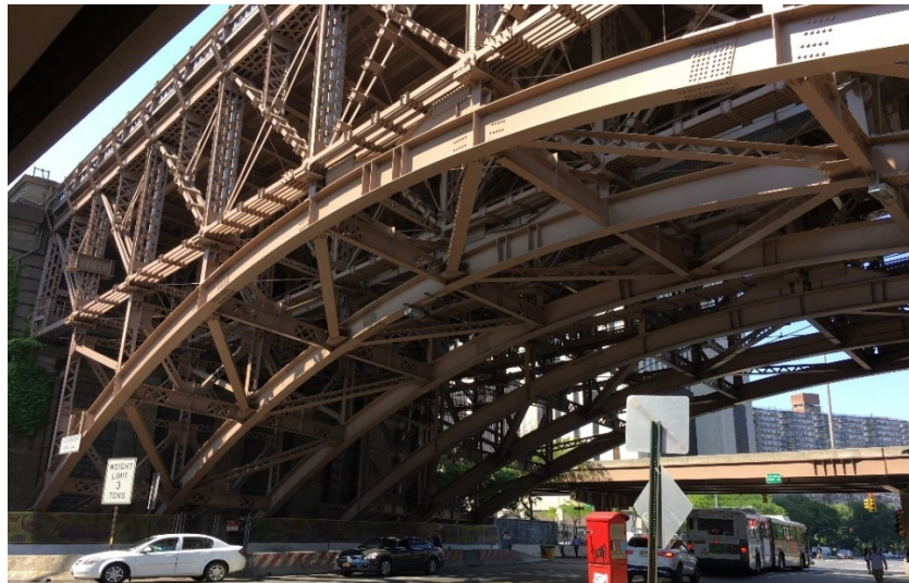
Figure 77. Photo. Retrofit of the Brooklyn Bridge with six arch systems.
