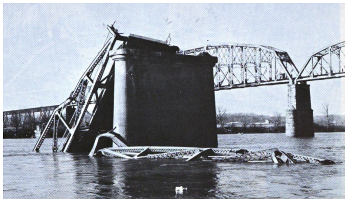
Figure 4. Photo. Silver Bridge collapse in 1967 (NTSB 1968).
