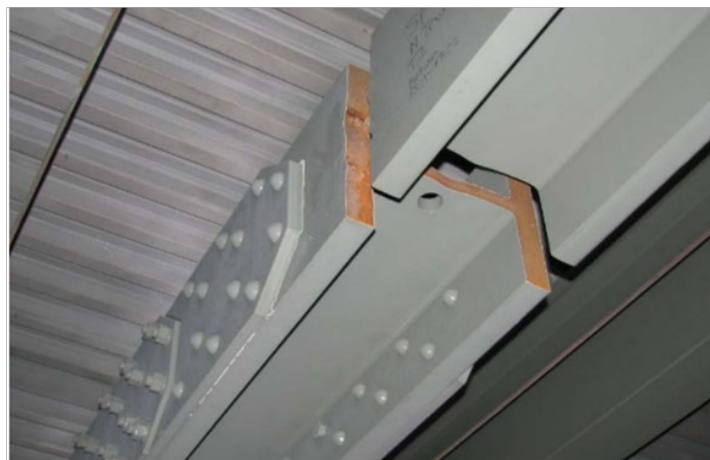
B. Close-up photo of the fractured member.
