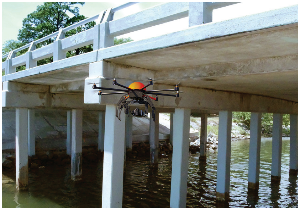
Figure 1. Use of UAS for in-service bridge inspection
