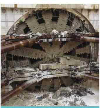
Figure 3. Photo. Tunnel boring machine cutter head breaking through final section of construction. ©Washington State Department of Transportation.
