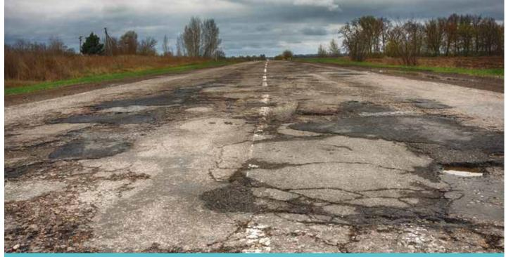
Figure 7. Photo. Example of severe pavement surface cracks and spiraling caused by weather conditions and vehicle weight wear and tear over time. ©undefined/iStock.
