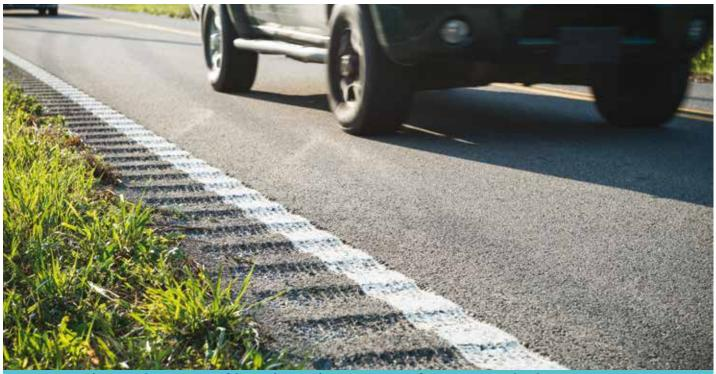
Figure 6. Photo. Pattern of depressions cut into pavement surface creates sound and vibration to alert drivers who are drifting out of the travel lane. ©Joel Carillet/iStock.
