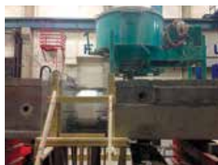
Casting of beam splice connection.
