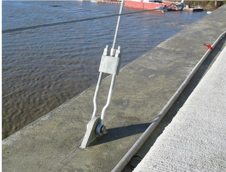
Figure 18. Photo. Anchorage attaching the line of crossies to the deck.
