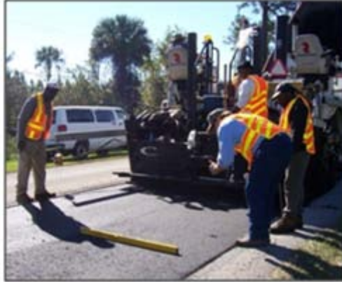
Figure 22. Photo. Placement of a high RAP mixture.
