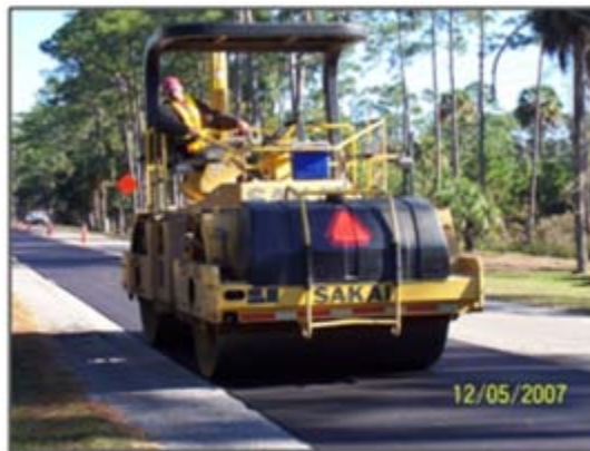
Figure 23. Photo. Compaction of a high RAP mixture.
