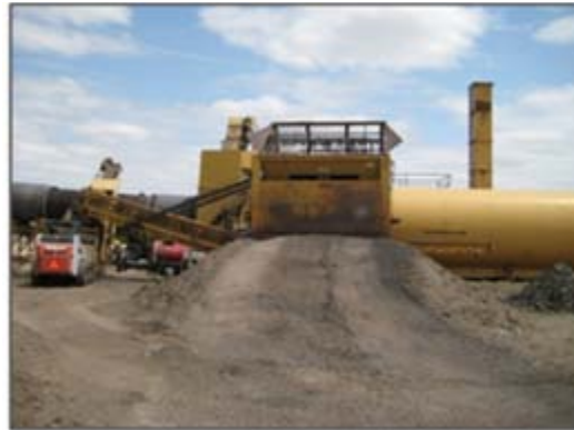
Figure 20. Photo. Scalping screen for RAP feed.
