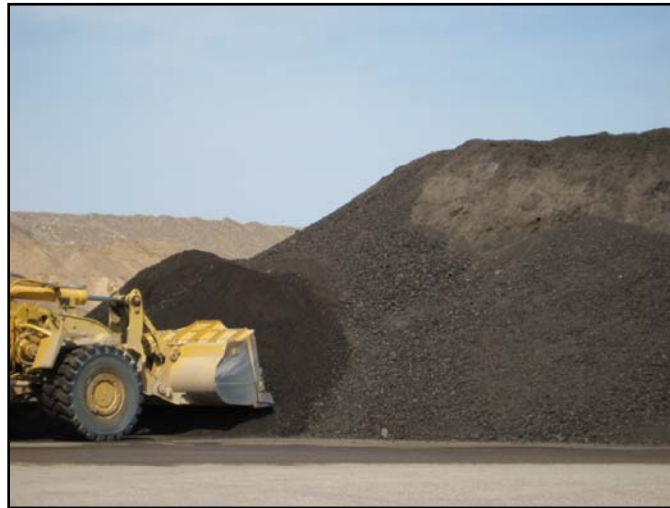
Figure 17. Photo. RAP stockpile being maintained.
