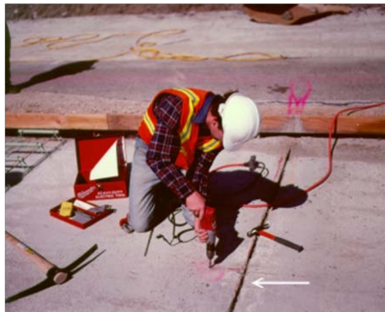
Figure 125. Photo. Cutting grooves in cement-treated base for instrument leads. (4)
