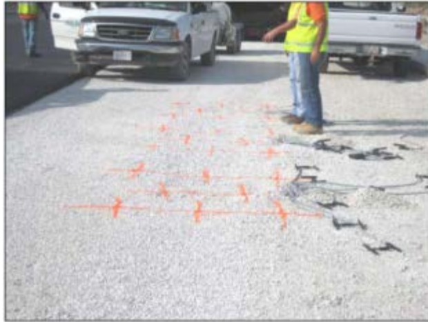
Figure 120. Photo. Marking the proposed locations of the gauges.
