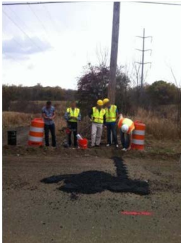
Figure 167. Photo. Installed prototypes ahead of the compactor.
