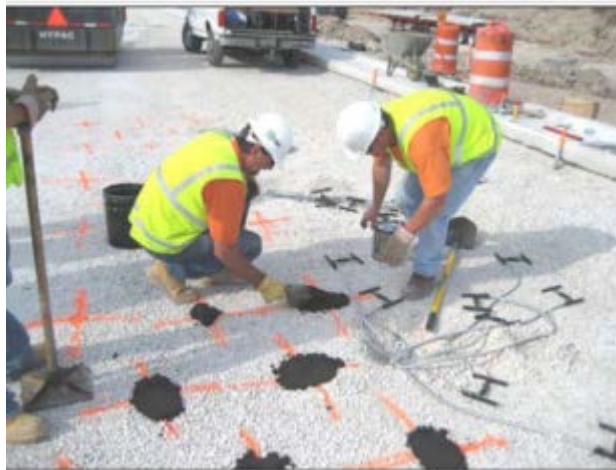
Figure 121. Photo. Placing sand/binder pad and fitting gauges. (3)
