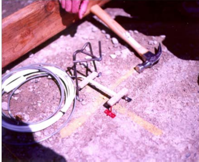
Figure 126. Photo. Collecting a concrete strain gauge using steel frames. (4)
