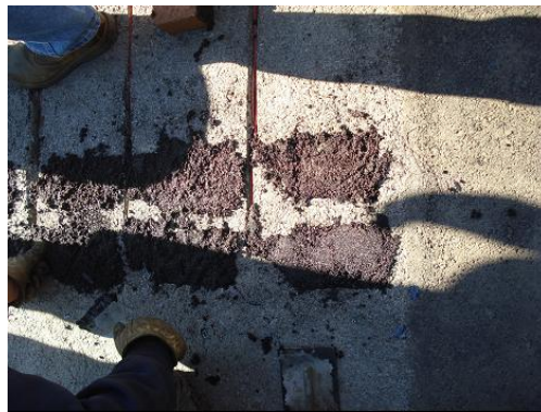
Figure 163. Photo. Installed prototypes.
