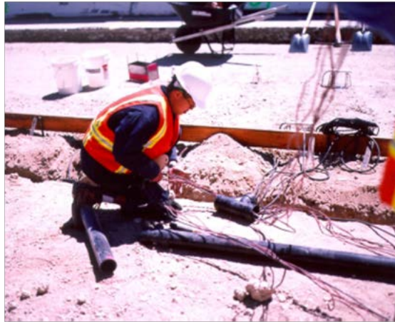
Figure 124. Photo. Laying instrument wiring and piping in aggregate base.
