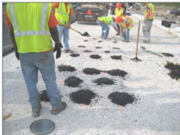
Figure 122. Photo. Placing screened asphalt on top of gauges and carefully compacting.
