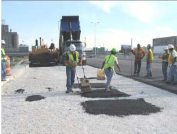
Figure 123. Photo. Compacting the unscreened asphalt over the gauge arrays.
