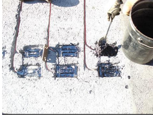
Figure 162. Photo. Special epoxy used to bond gauges to surface.
