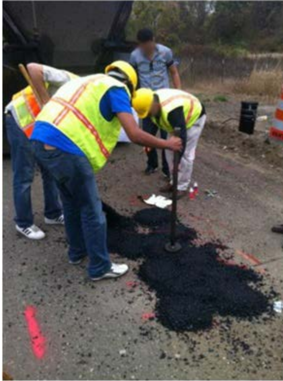
Figure 166. Photo. Manual compaction of HMA patches.
