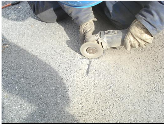
Figure 157. Photo. Grinding the existing pavement before bonding gauges to the surface.
