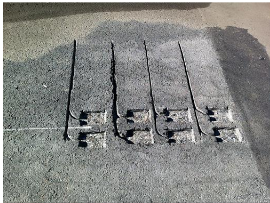
Figure 161. Photo. Prepared grooves for prototype installation.
