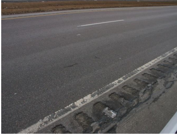
A. View of first stage—occurrence of short longitudinal cracks in and/or adjacent to the wheel path.
