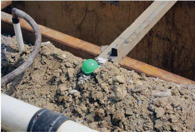
Figure 3. Photo. RFID marker next to a trench.
