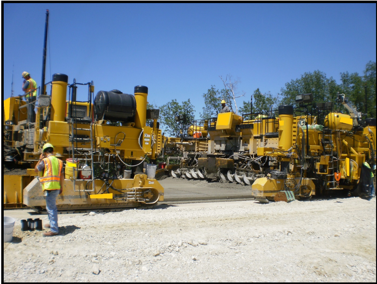
Figure 35. Photo. Concrete AMG paving operation controlled with total stations on rural remote site on U.S. Route 50 (east of Jefferson City, MO).
