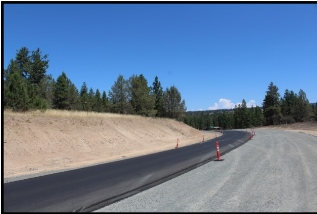
Figure 4. Photo. Crushed stone base for asphalt pavement placed with AMG equipment.
