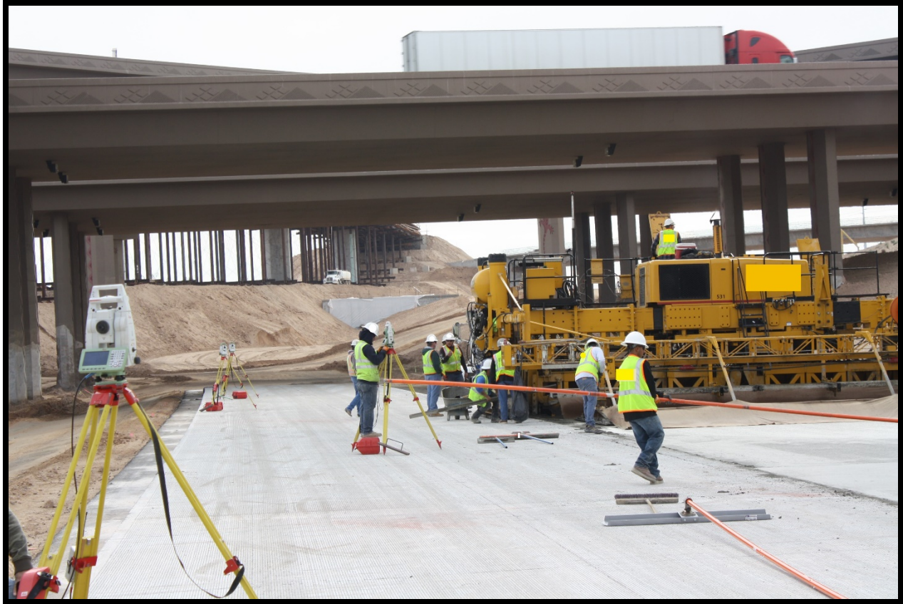
Figure 69. Photo. Robotic total station-guided concrete paver.
