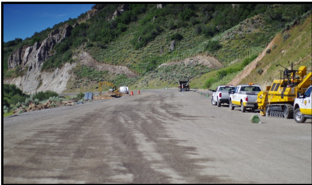
Figure 2. Photo. AMG grade control for subsequent asphalt paving often stops at the top of the granular subbase. (8)
