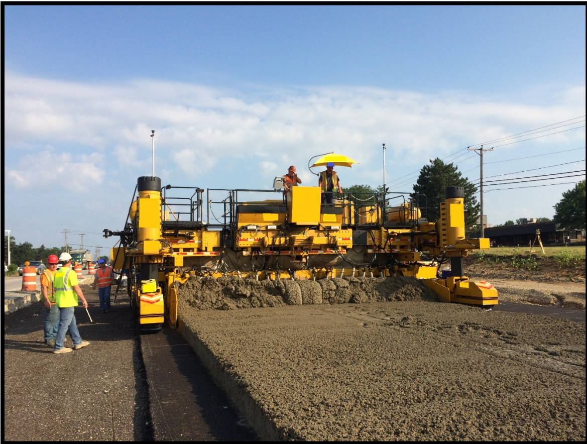
Figure 21. Photo. Concrete AMG paving operation controlled with total stations under live traffic on I-90 (Chicago metro area).
