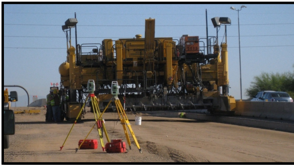
Figure 18. Photo. Concrete AMG paving operation controlled with total stations under live traffic on Arizona Loop 101 (Phoenix metro area).
