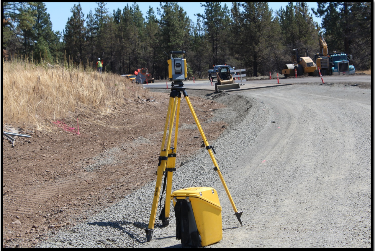
Figure 51. Photo. Total stations are used for checking the grade and confidence points.
