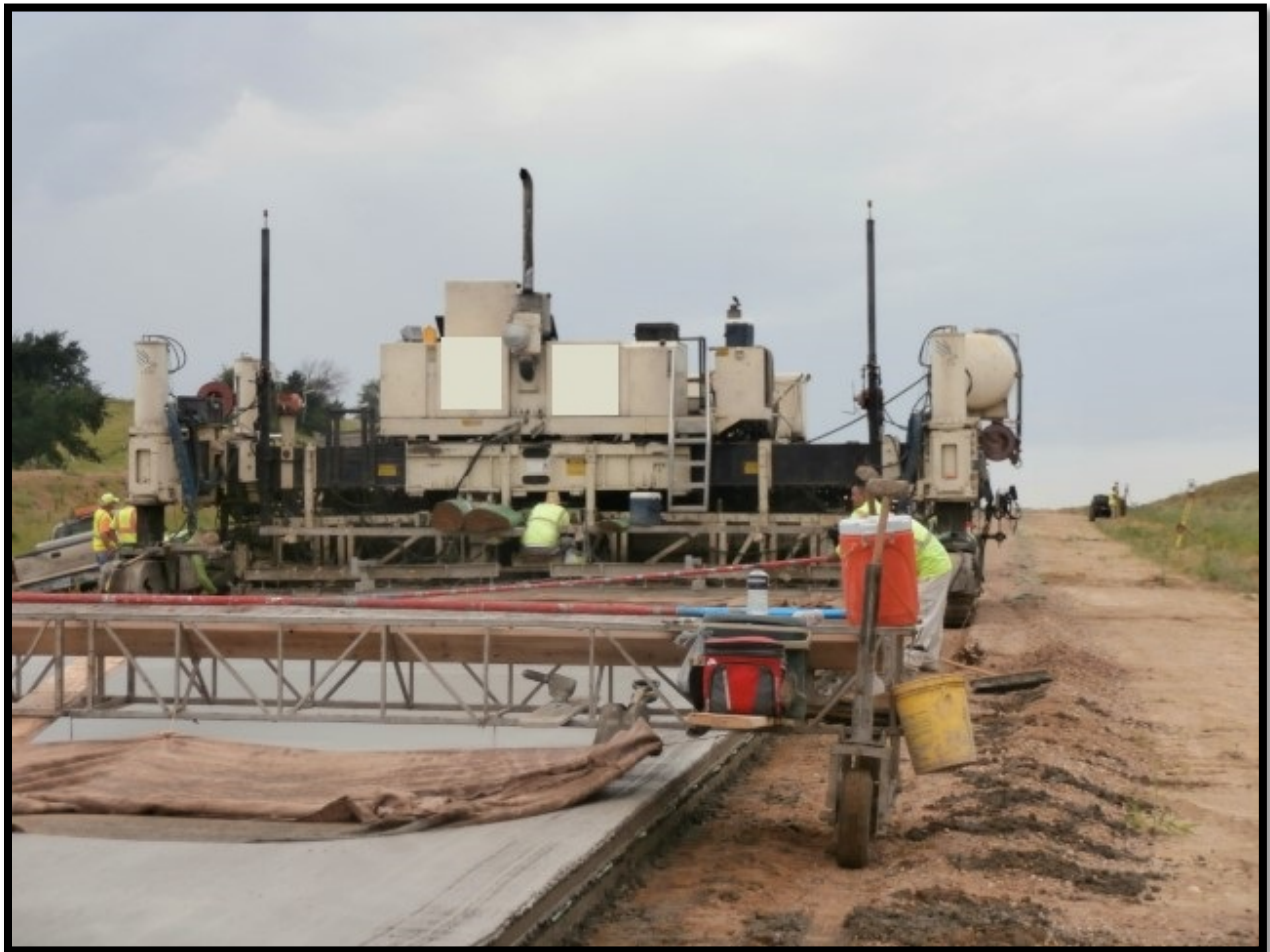
Figure 29. Photo. Concrete AMG paving operation controlled with total stations on rural remote site on U.S. Route 20 (east of Sioux City, IA).
