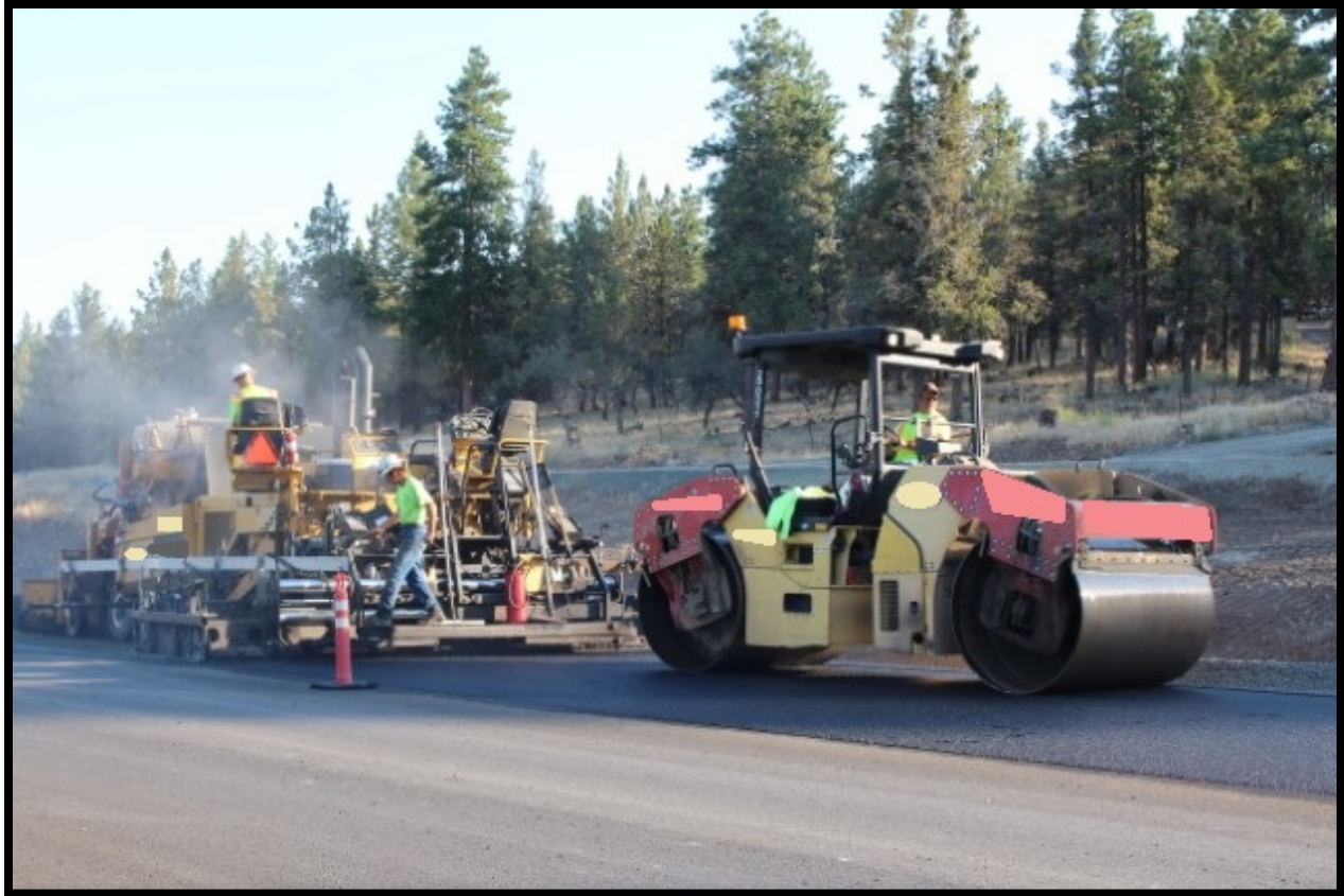
Figure 52. Photo. Asphalt paving equipment did not use AMG technology. All rough and fine grading used AMG equipment (GPS technology).
