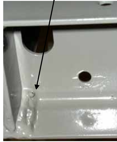
Subassembly bottom joint reinforced weld
