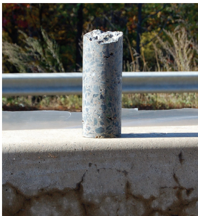
Figure 4. Closeup of an extracted core from a concrete barrier.
