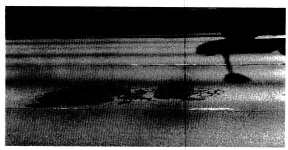
Figure 11. Bituminous patch in existing CRCP.
