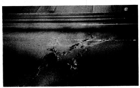
Figure 12. Close-up of crack spalling.
