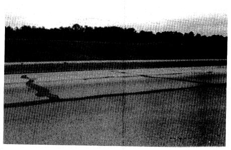
Figure 35. Reflection crack in AC-overlaid CRCP.
