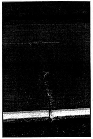
Figure 10. Extra wide crack in existing CRCP.
