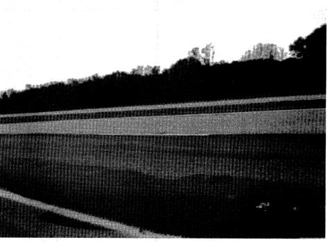
Figure 36. A typical rut in AC overlay of CRC pavement.
