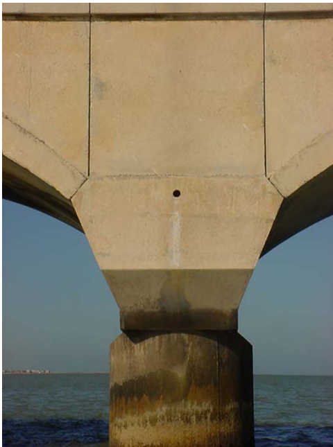
Figure 24. Photograph of hinged arches and piling.
