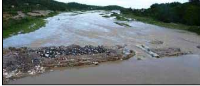
Figure 29. Photo. Temporary Roadway over the River.
