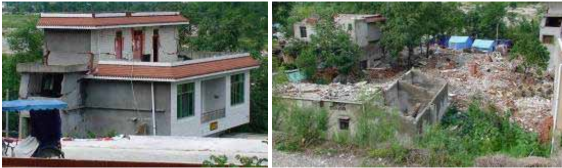
Figure 33. Photo. Building Damage in Nearby Town.
