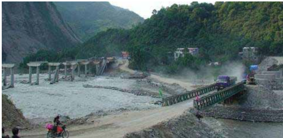
Figure 49. Photo. Overview of Temporary Bridge Construction.
