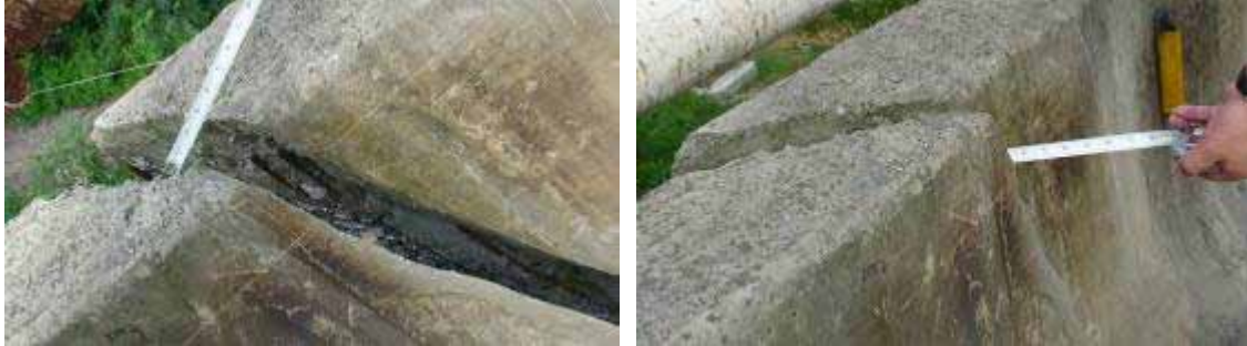
Figure 32. Photo. Measurement of Expansion Joint Offset.
