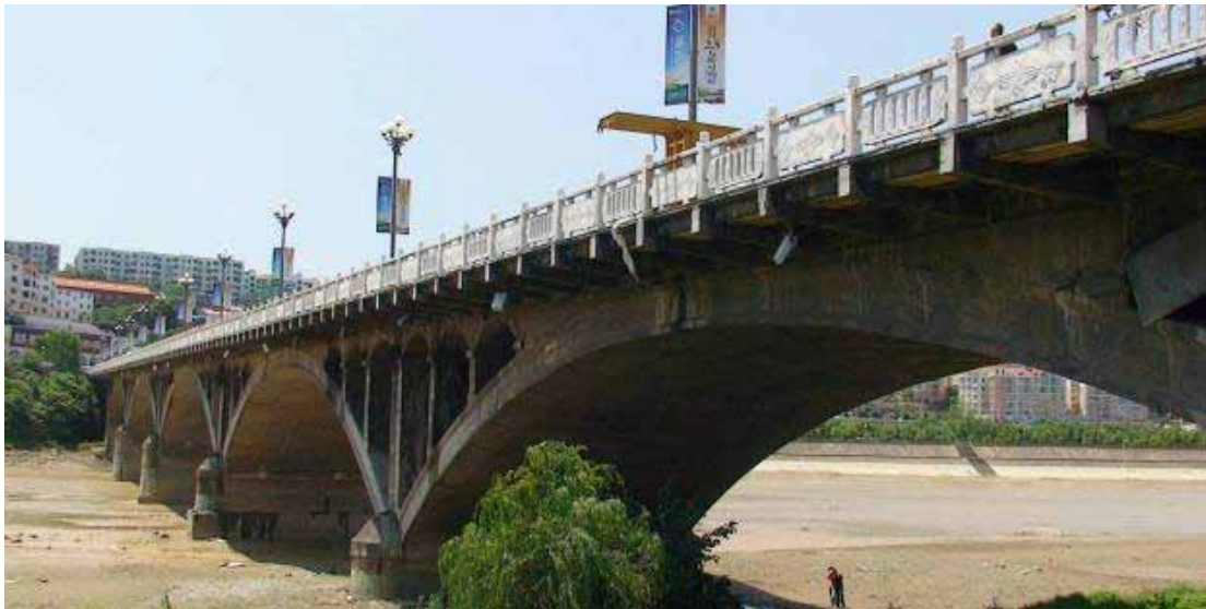
Figure 38. Photo. Overview of Nanhe Bridge.
