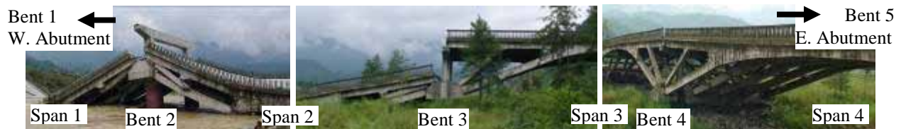
Figure 17. Photo. Overall View of the Remaining Arches.
