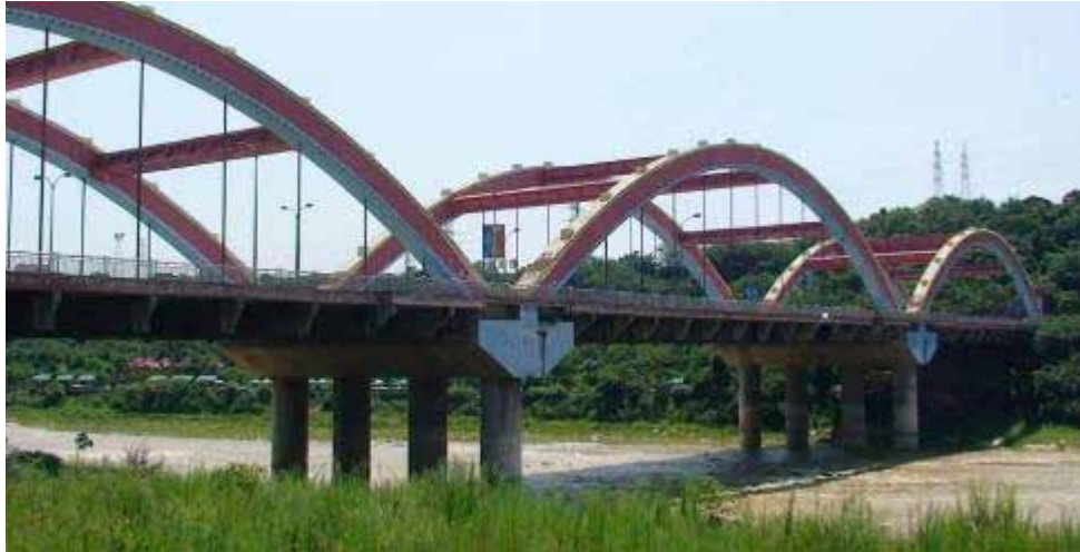
Figure 34. Photo. Overview of Baiyun Bridge.
