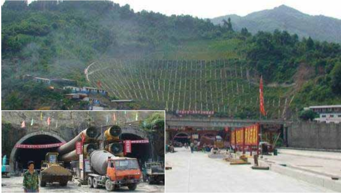
Figure 53. Photo. Miaozihiping Tunnel.
