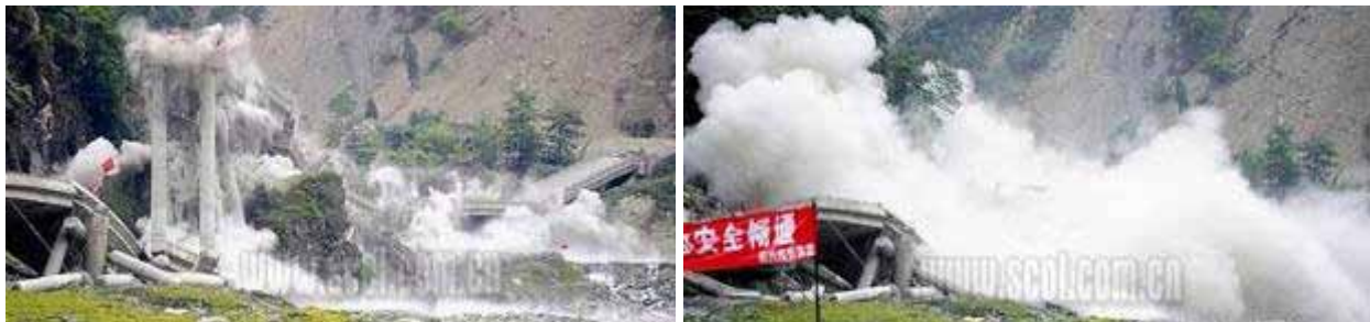
Figure 70. Photo. Blast Demolition of Baihua Bridge.
