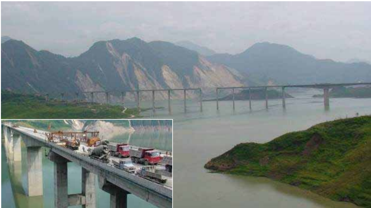
Figure 54. Photo. Overview of Miaozihiping Bridge.
