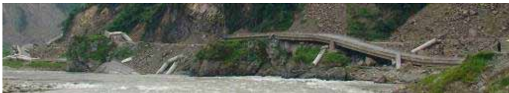
Figure 71. Photo. After Demolition of Baihua Bridge.
