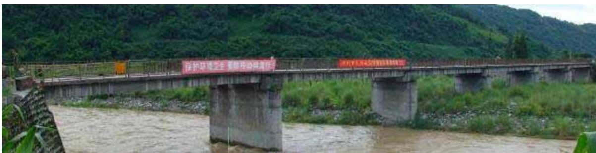
Figure 9. Photo. Overview of Zhima Bridge.
