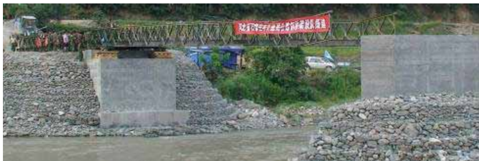
Figure 50. Photo. Bailey Bridge in Place.
