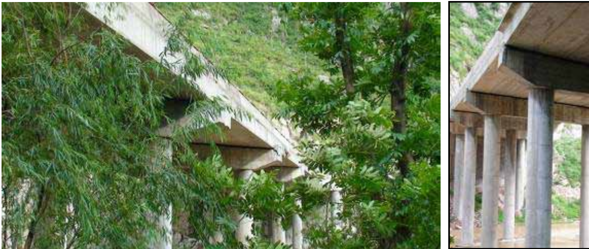
Figure 30. Photo. Overview of Baimayan Bridge.
