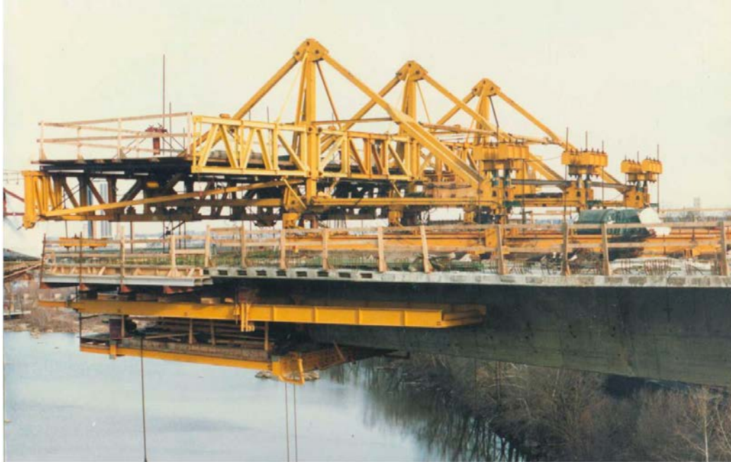
Figure 14. Photo. CIP balanced cantilever bridge during construction using form traveler.
