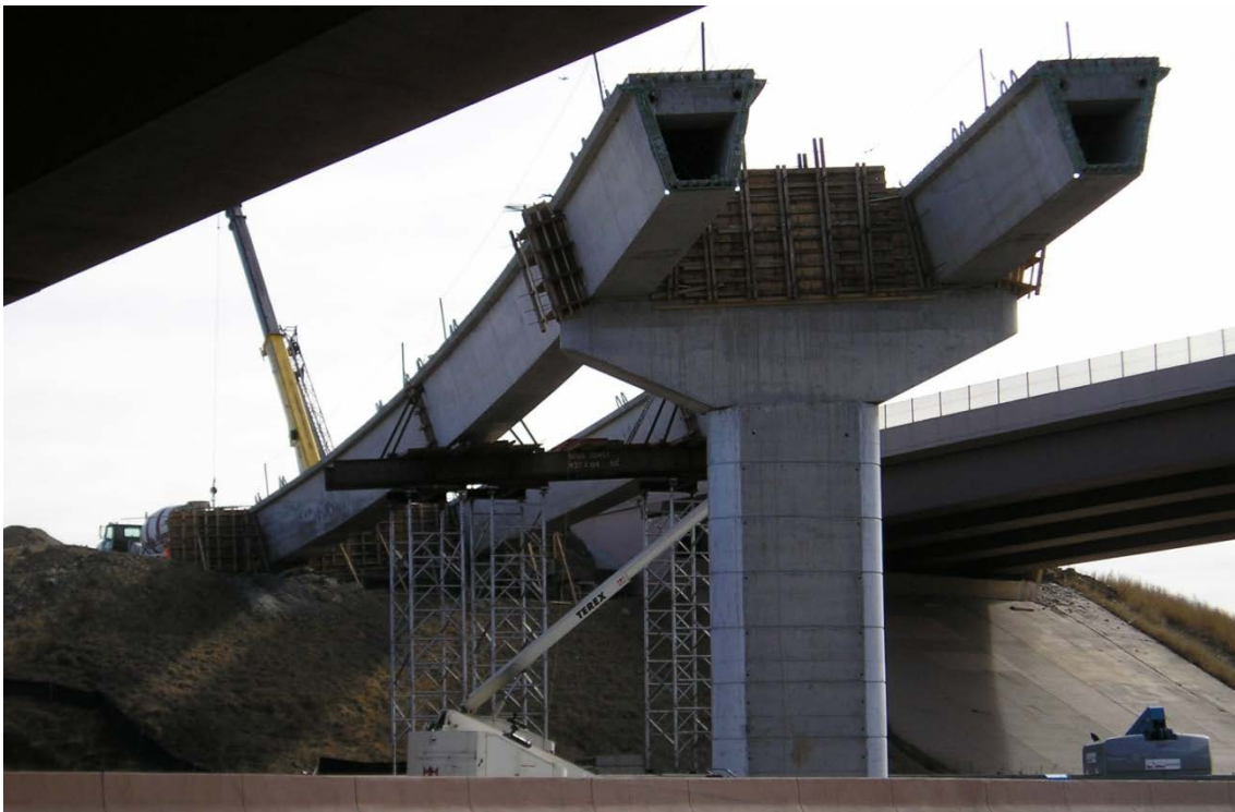
Figure 20. Photo. Precast spliced U-girder bridge during erection.
