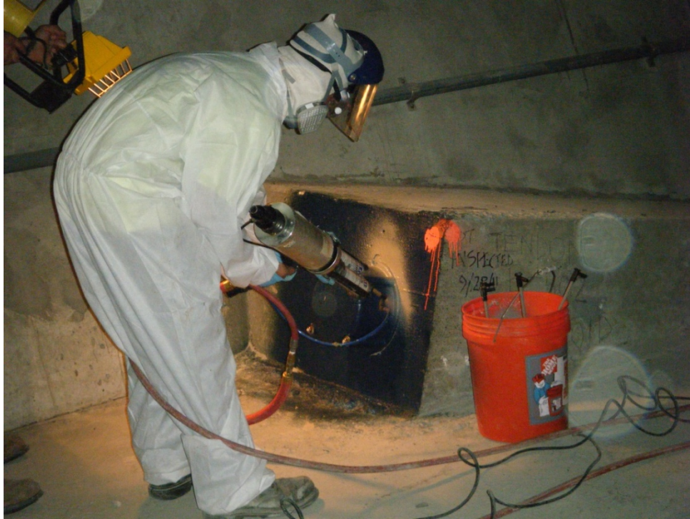
Figure 77. Photo. Applying elastomeric coating over a grout cap.
