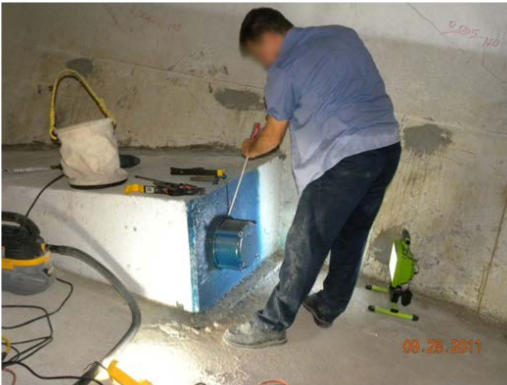
Figure 62. Photo. Removing a permanent grout cap.
