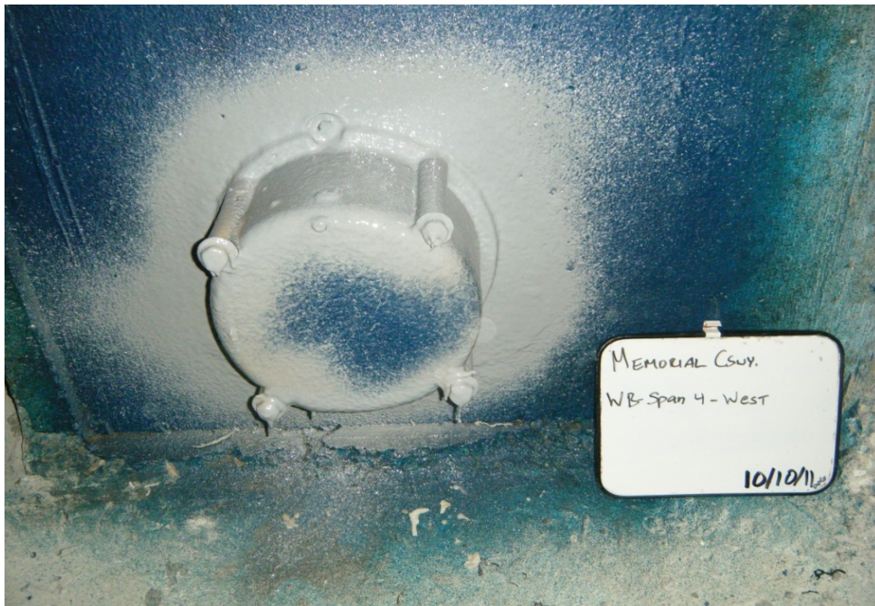
Figure 77. Photo. Applying elastomeric coating over a grout cap.
