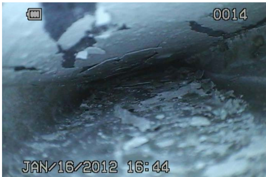
Figure 58. Photo. View of a duct interior revealing a channel air void.
