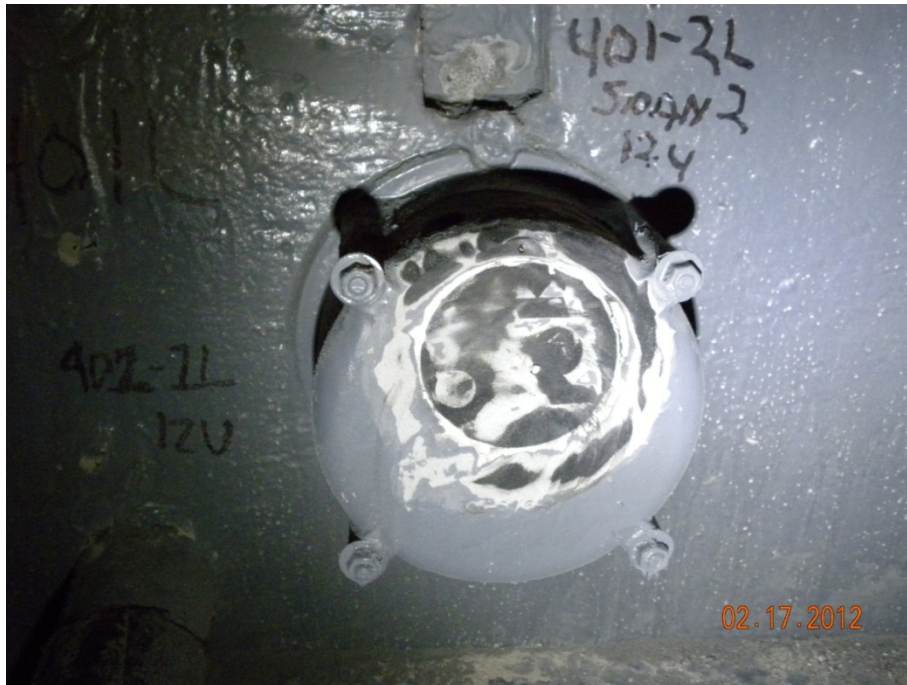
Figure 76. Photo. Completed restoration of a partially cut grout cap prior to coating.
