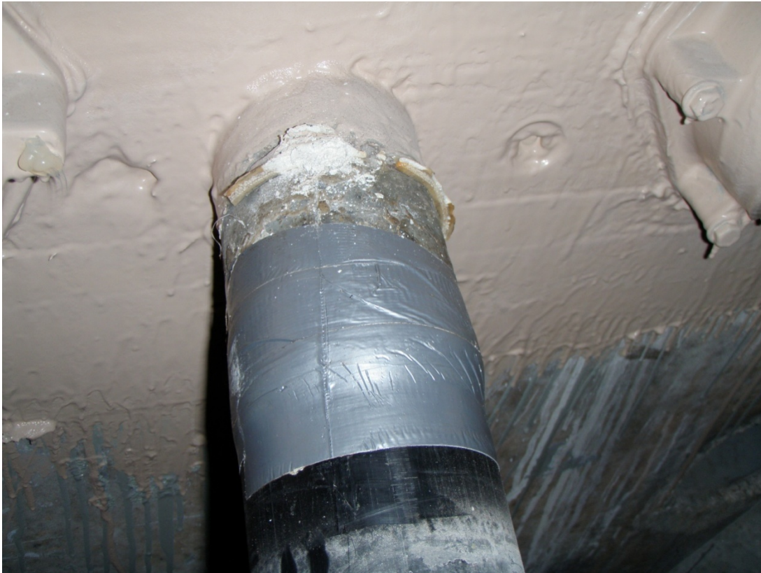
Figure 73. Photo. Temporary restoration of an external tendon.
