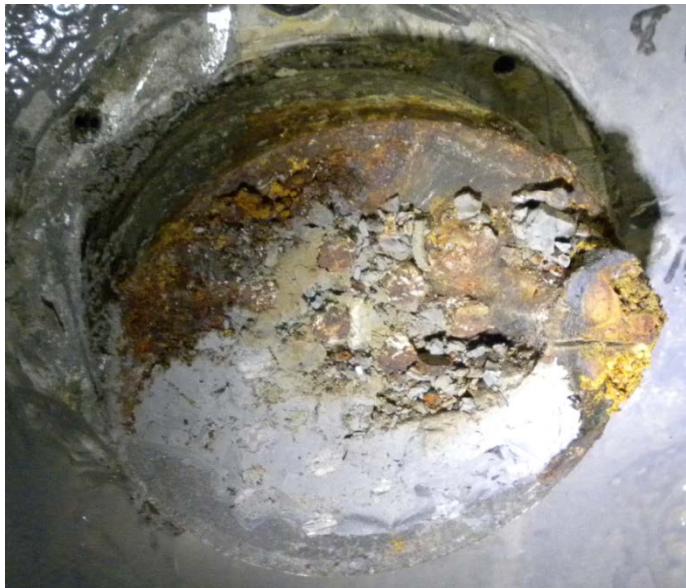
Figure 31. Photo. Opened tendon end showing types 3 and 1 grout and strand corrosion products.
