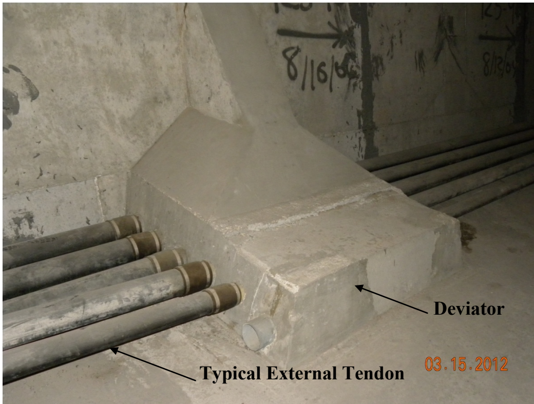
Figure 6. Photo. External tendons at deviator.
