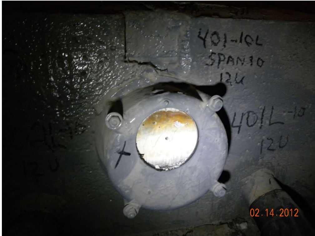
Figure 65. Photo. Partial removal of a grout cap.
