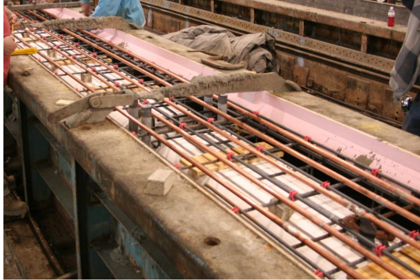
Figure 20. Photo. Copper tubes in the box beam prior to casting.
