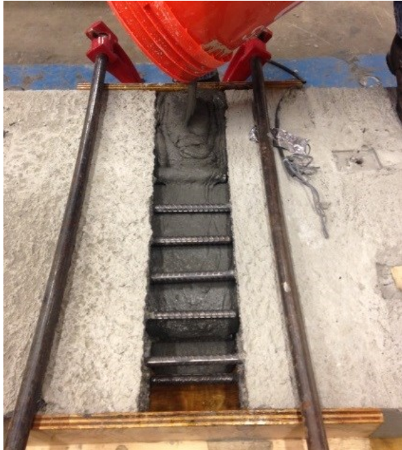
Figure 25. Photo. Placement of UHPC in the connection region of a deck-level connection specimen.
