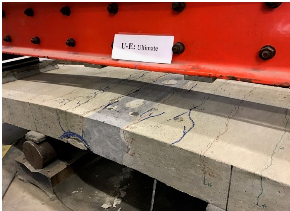
Figure 184. Photo. Specimen U-E after ultimate loading.
