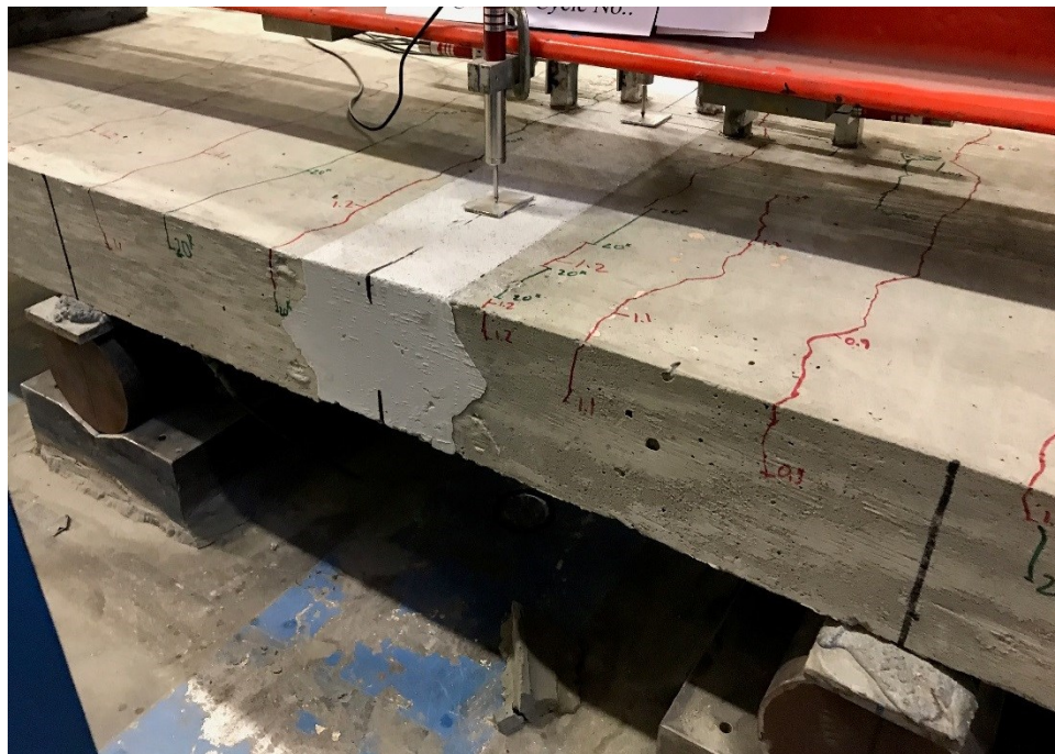
Figure 175. Photo. Observed cracking in specimen U-D after fatigue loading.
