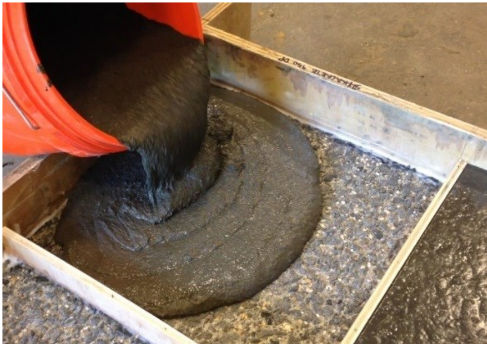
Figure 24. Photo. Placement of UHPC topping on interface bond test specimens.
