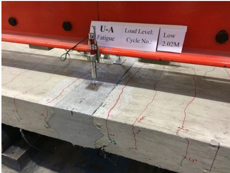
Figure 172. Photo. Observed cracking in specimen U-A after fatigue loading.
