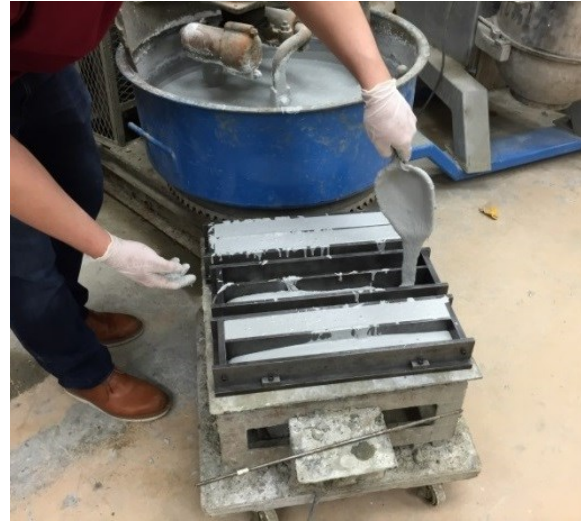
Figure 23. Photo. Placement of UHPC in a prismatic specimen.
