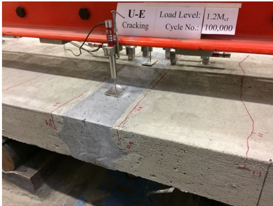
Figure 168. Photo. Observed cracking in specimen U-E after pre-cracking cyclic loading.
