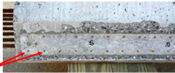
Figure 7. Illustration. Compound Figure Showing DEMEC Points on Girder End.
