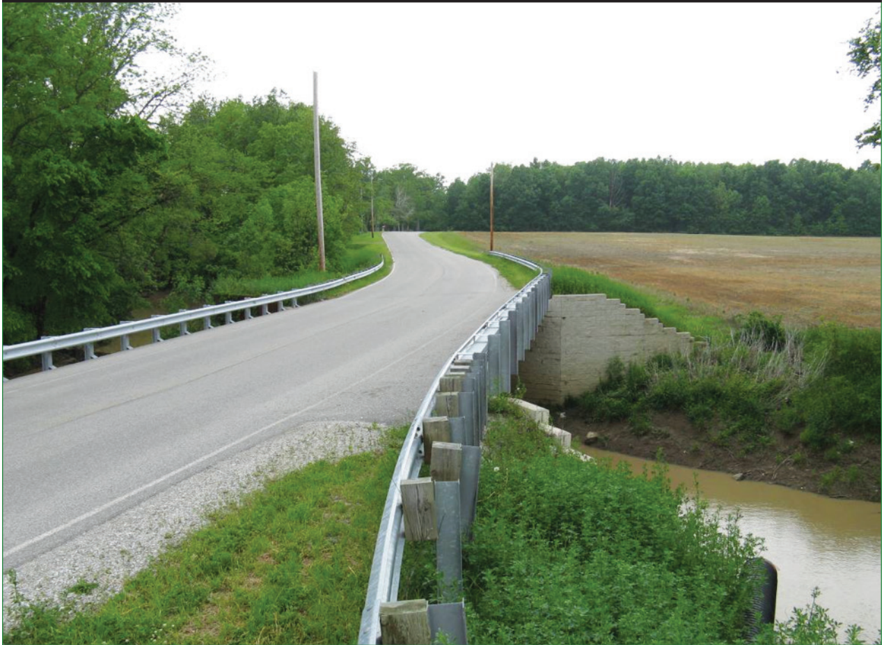
Figure 1. Photo. Bowman Road Bridge—the first GRS-IBS.
