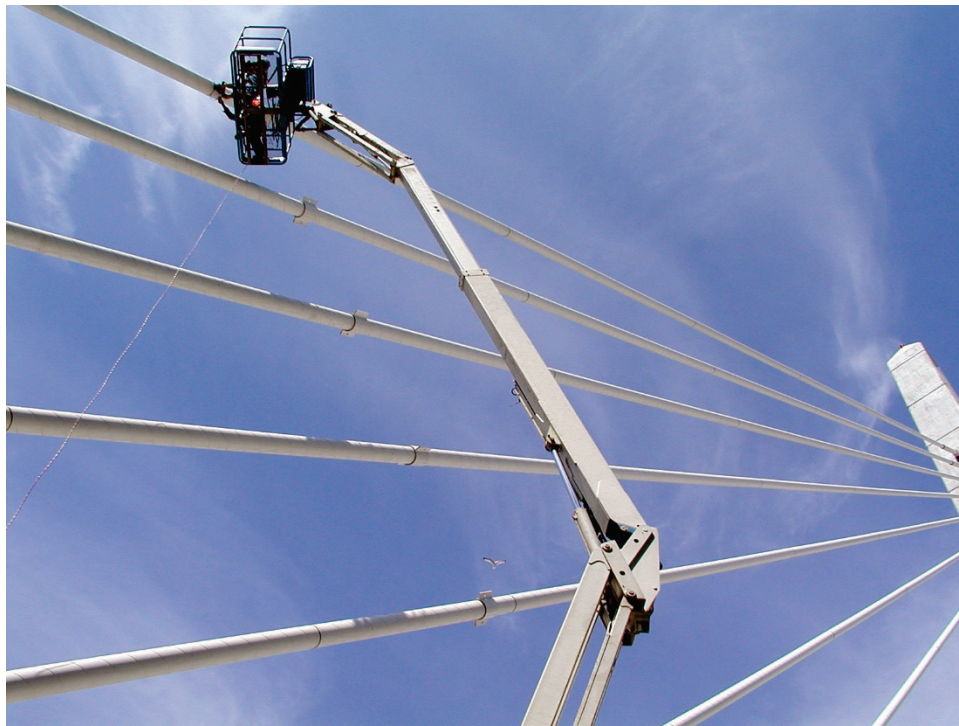
Figure 17. Photo. Installation of accelerometer on a stay cable.
