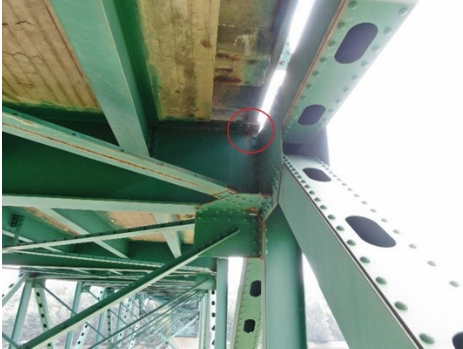
Figure 49. Photo. Defect location as seen from a UBIT.
