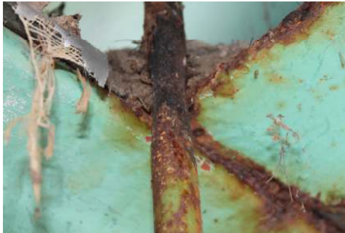
Figure 56. Photo. Image of steel hanger rod taken by inspector using handheld camera.
