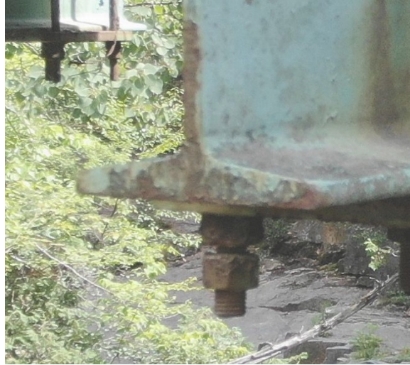
Figure 61. Photo. Enlarged UAS image of backed off nut on hanger rod.
