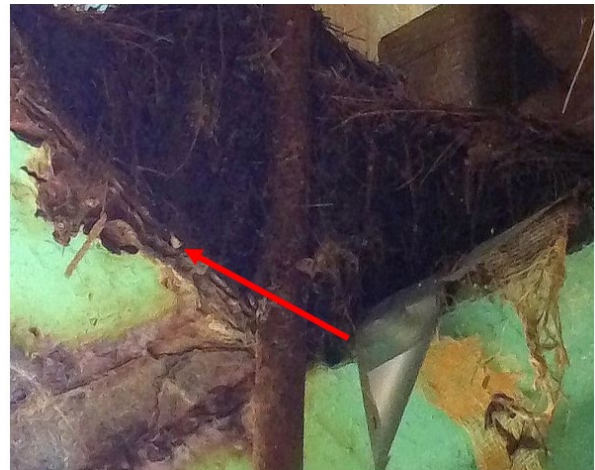
B. Zoomed photo showing section loss.
