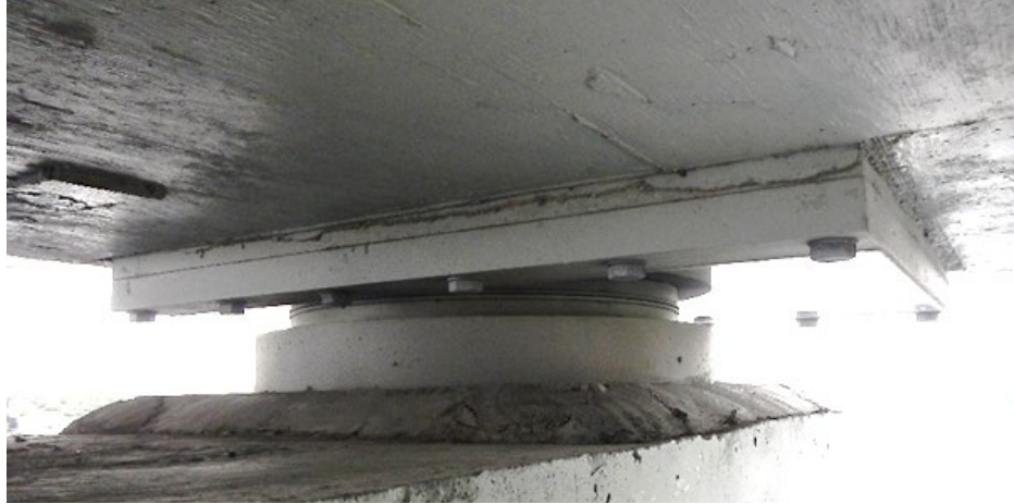
Figure 44. Photo. Image of bearing taken with handheld camera from the staging on the underside of the bridge.
