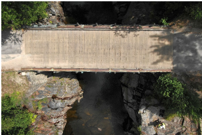
Figure 58. Photo. Overhead image of deck condition taken by a UAS.
