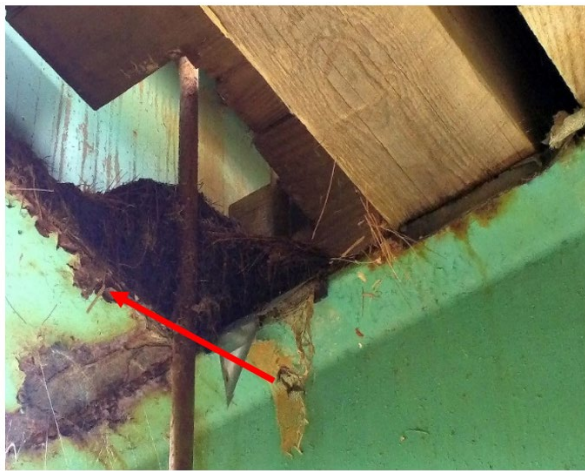
A. Nonzoomed photo showing section loss.
