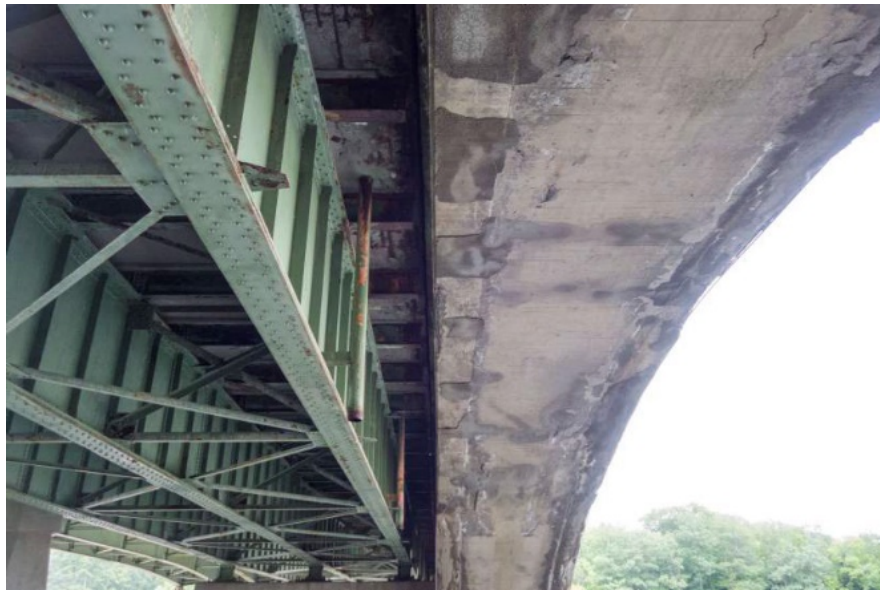
Figure 23. Photo. Typical underside view of concrete arch, inaccessible using a UBIT for imaging.
