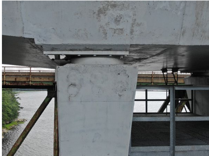
Figure 45. Photo. Raw image of the pier 8 bearing.
