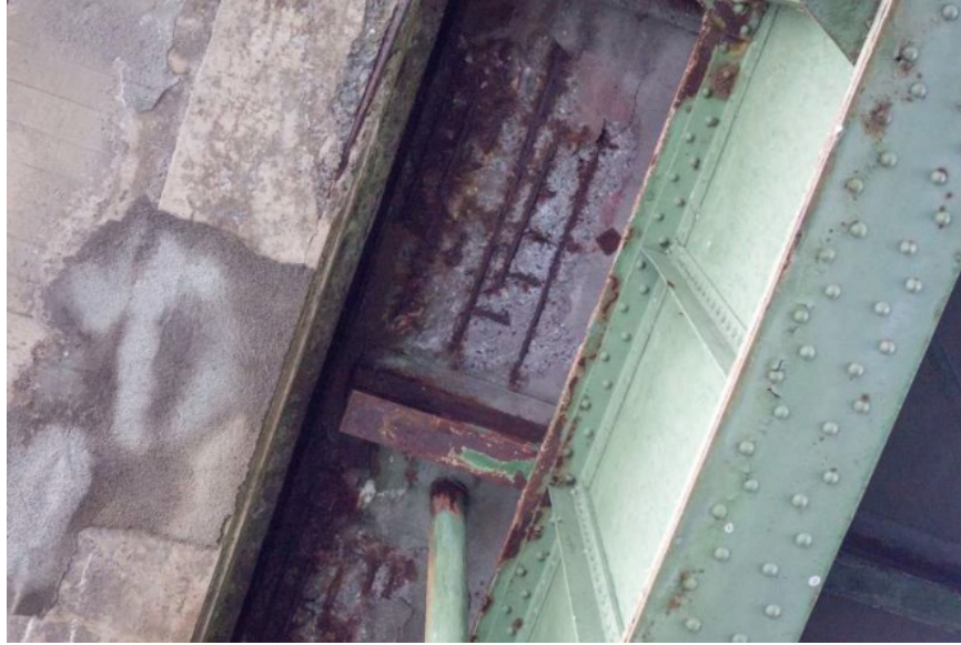
Figure 24. Photo. Image of the underside of concrete arch between the steel girders using an upward facing camera on the UAS.
