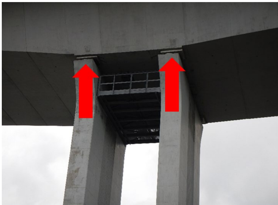
Figure 43. Photo. Image of Sagadahoc Bridge piers 8 and 9 bearings captured by UAS.
