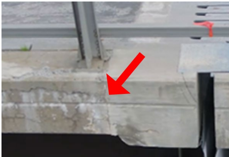
Figure 41. Photo. Snapshot from 4K video showing the joint, curb, and cracking on the fascia.
