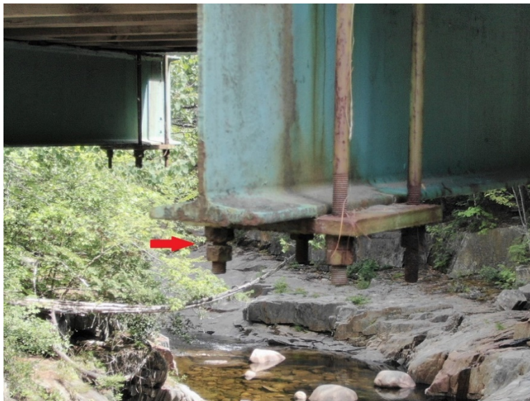
Figure 60. Photo. UAS image of backed off nut on hanger rod.
