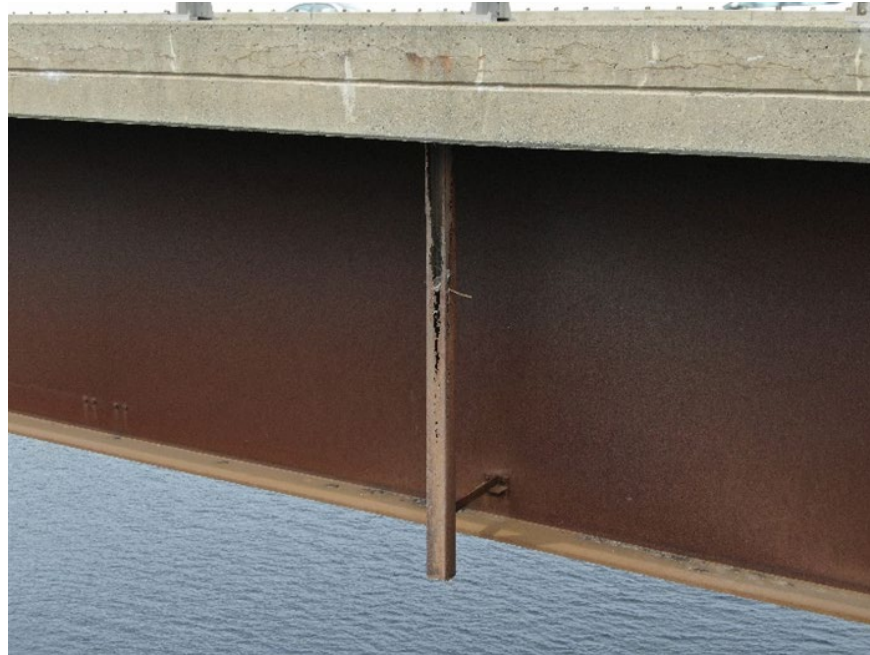
Figure 38. Photo. UAS image of defective downspout.
