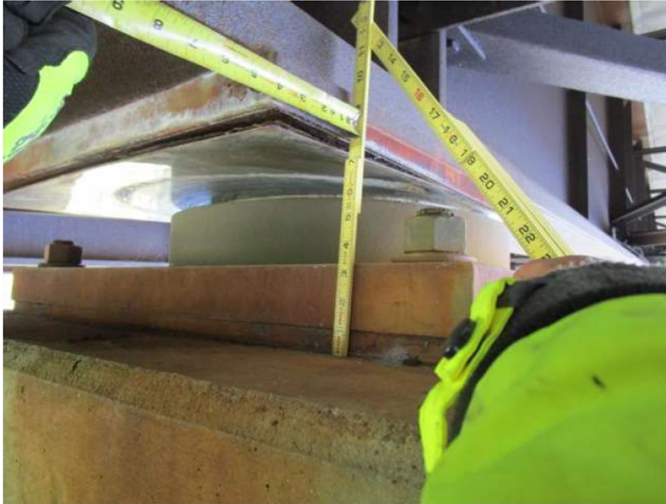
Figure 35. Photo. Inspector measuring bearing shift.
