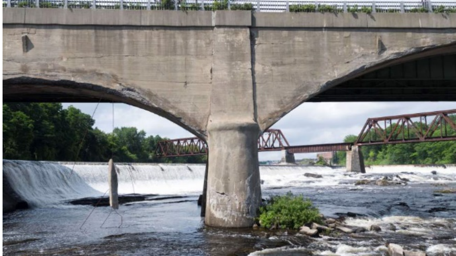
Figure 22. Photo. UAS-captured downstream view of pier and spalled concrete hanging from span.
