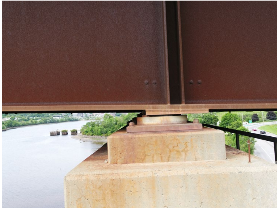
Figure 36. Photo. UAS image showing bearing out of alignment.
