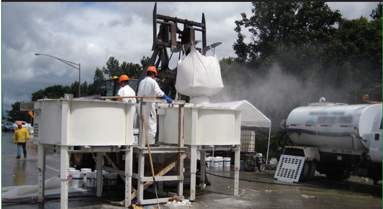
Figure 27. Photo. Mixing operation for the field-cast UHPC. (25)
