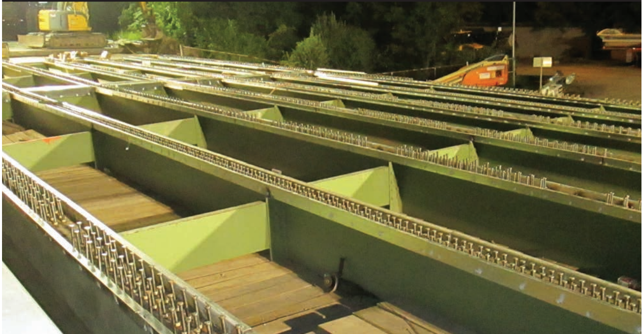
Figure 19. Photo. Superstructure prepared for precast panel installation. (25)
