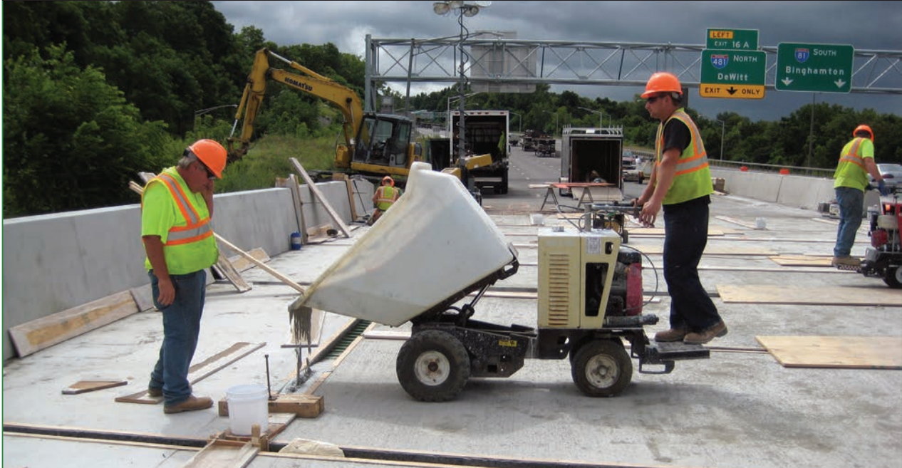
Figure 28. Photo. Placing operation for the field-cast UHPC. (25)
