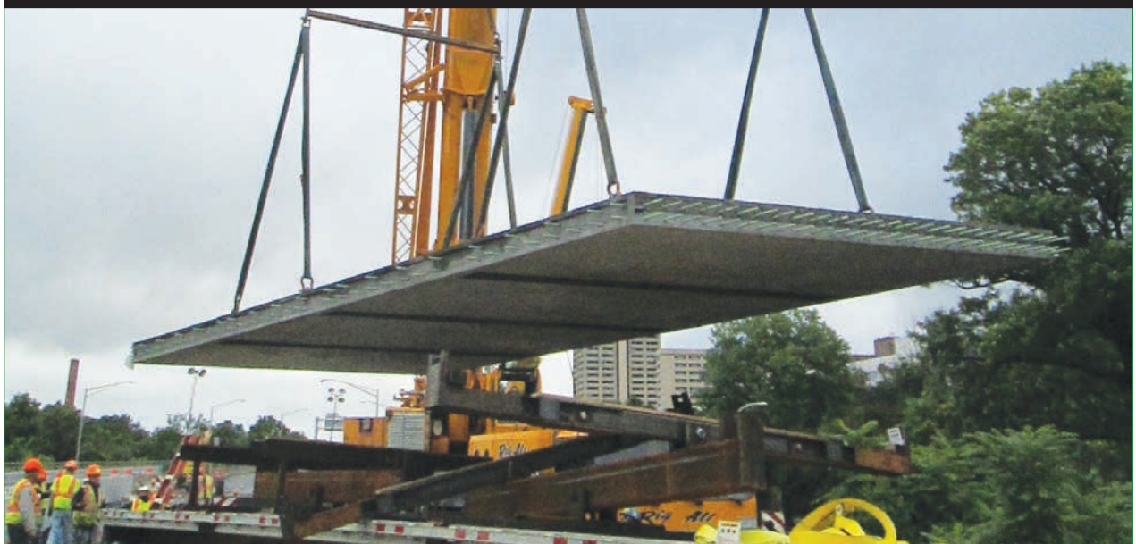
Figure 20. Photo. Transport and rigging of precast deck panel. (25)
