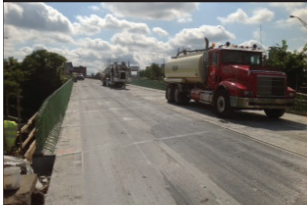
Figure 18. Photo. Surface profiling of a bridge deck on I-81 near Syracuse, NY.
