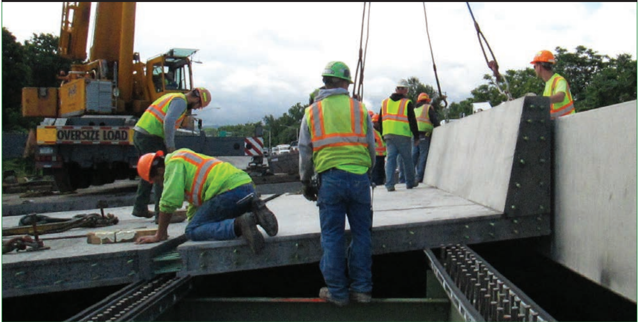
Figure 21. Photo. Installation of precast panel with integral barrier. (25)
