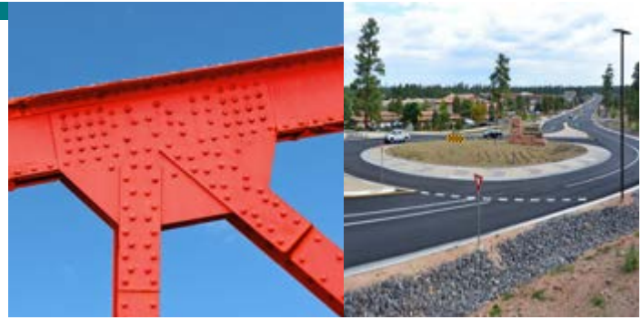
Left: Gusset plate. Source: FHWA. Right: Roundabout. Source: Photo by Michael Quinn / CC BY 2.0
