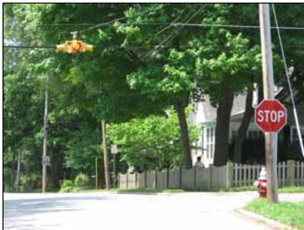
Figure 1. Photo. Example of Standard Overhead Flashing Beacon.
