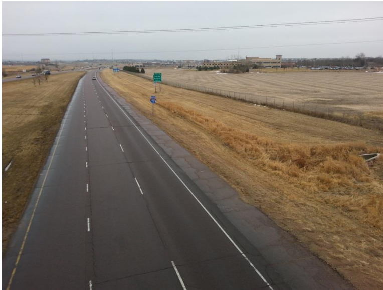
Figure 20. Photo. Left-hand acceleration lane terminating in a lane-reduction taper.
