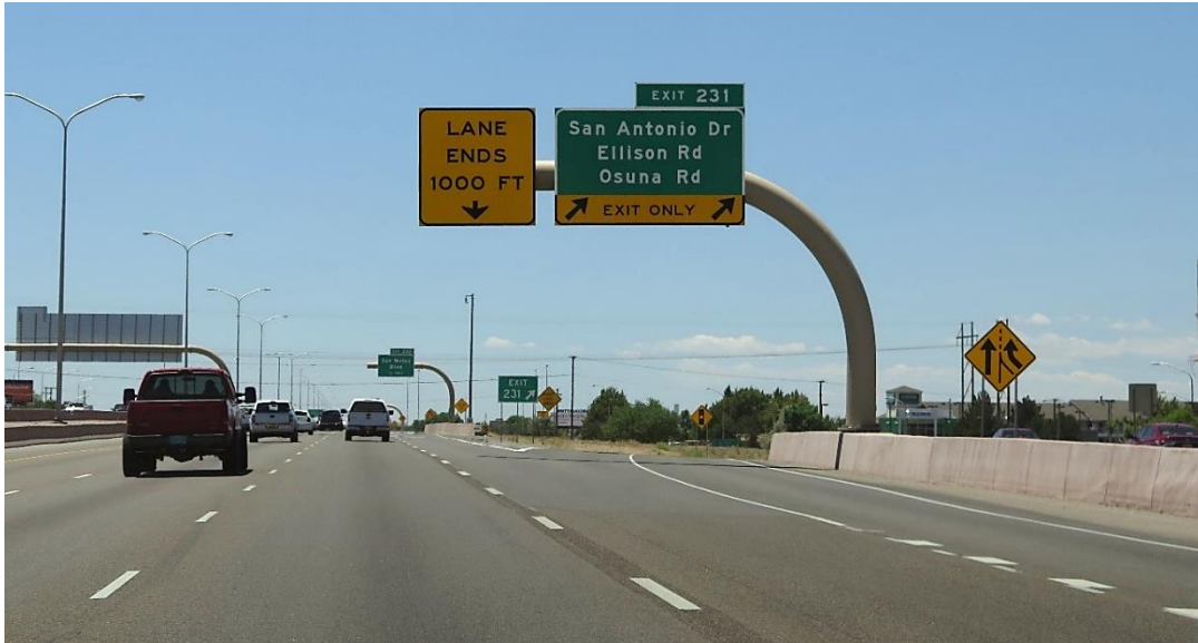
Figure 14. Photo. Escape lane signing that does not adhere to the consistency principle because the continuing lane is signed as an exit-only lane.
