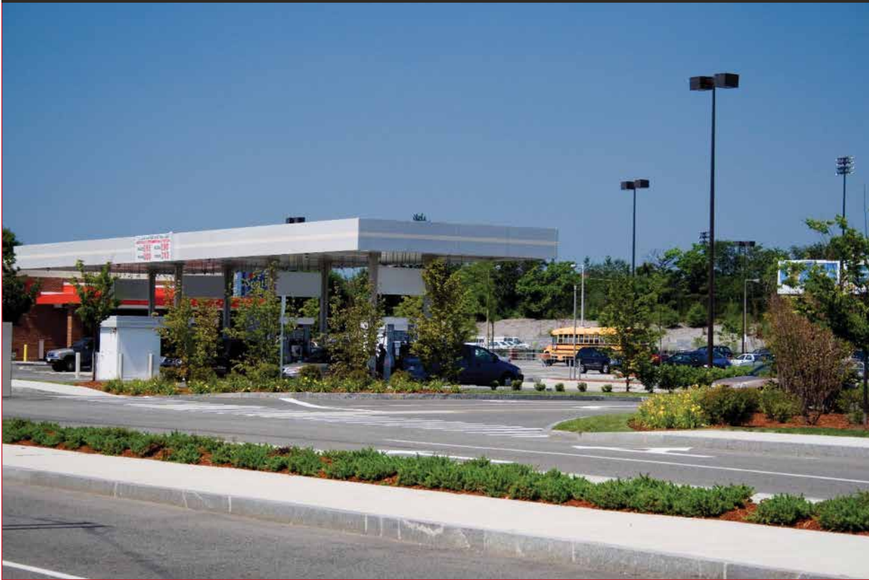
Figure 1. Photo. RIRO stop-controlled intersection.
