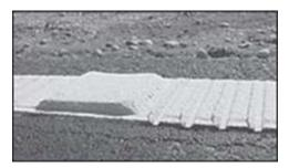
Figure 1. Photo. Raised profiled thermoplastic marking.<sup>(1)</sup>
