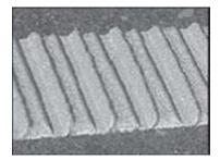
Figure 2. Photo. Inverted profiled thermoplastic marking.<sup>(1)</sup>
