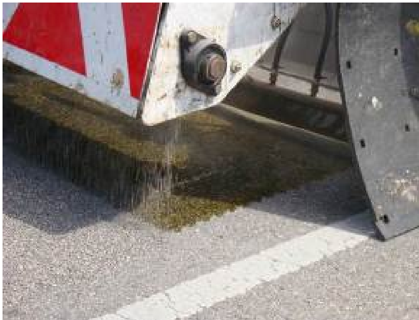
Figure 1. Photograph. Manual HFST installation.
