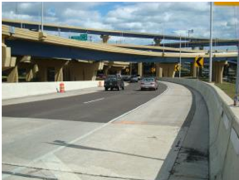
Figure 3. Photograph. HFST post installation.
