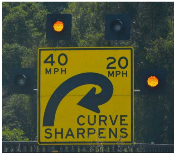
Figure 5. Photo. Advance curve and speed sign with Curve Sharpens text. (33)
