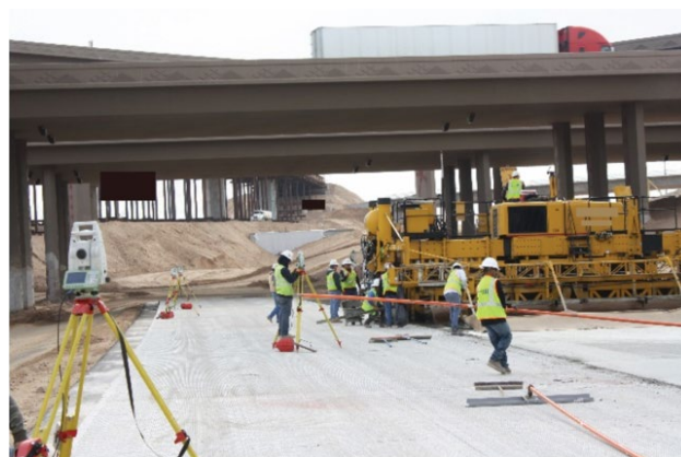
Figure 3. Photo. Total station-guided concrete paver.
