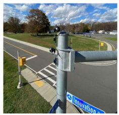
Figure 1. FLIR Camera at an intersection at the TFHRC.
