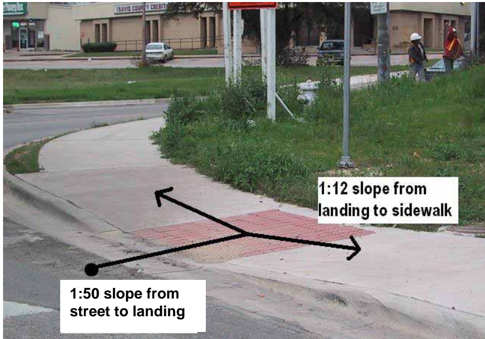
Figure 8-16. Photo. Parallel curb ramp.
