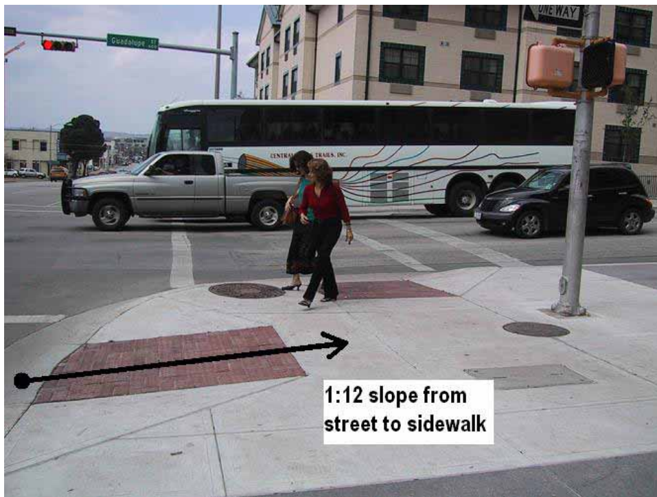
Figure 8-15. Photo. Perpendicular curb ramp.
