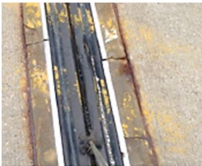
300 – Strip Seal Expansion Joints
