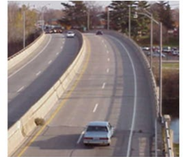
12 – Reinforced Concrete Deck
