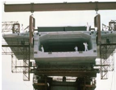
104 Prestressed Closed Web/Box Girder (Segmental)
