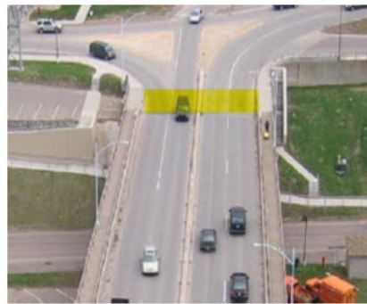
321 – Reinforced Concrete Approach Slabs
