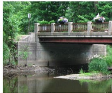
215 Reinforced Concrete Abutment
