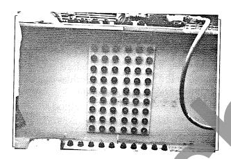
Snug tightening shall progress systematically from the most rigid part of the connection to the free edges, and then the bolts of the connection shall be retightened in a similar systematic manner as necessary until all bolts are simultaneously snug tight and the connection is fully compacted.
