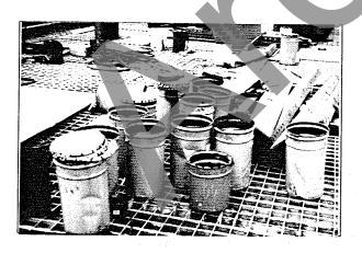
Fasteners shall be protected from dirt and moisture at the job site. Only as many fasteners as are anticipated to be installed and tightened during a work shift shall be taken from protected storage. Fasteners not used shall be returned to protected storage at the end of the shift.
