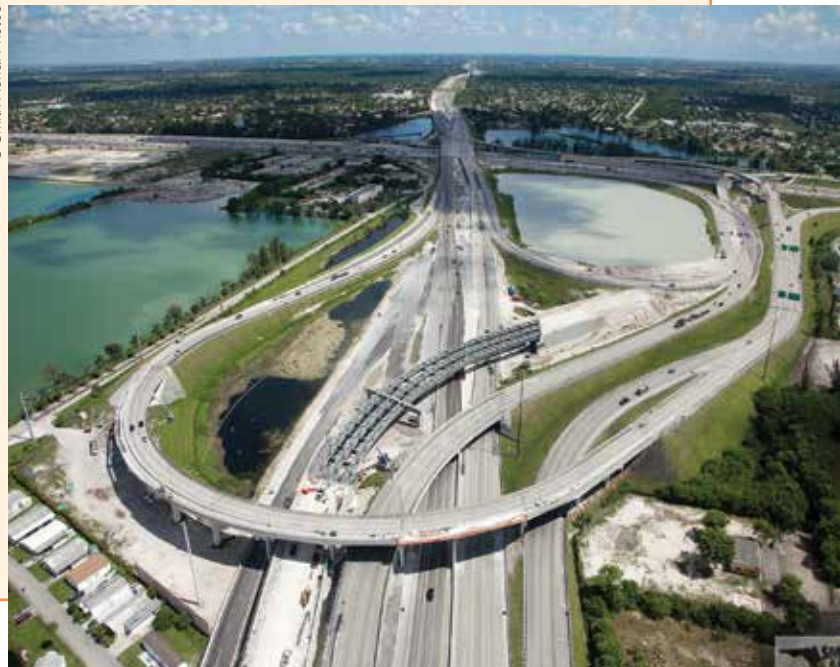
Interstate 595 and Florida Turnpike interchange
