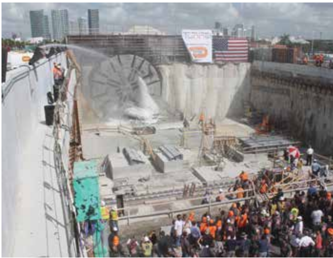
Celebration of the arrival of the Tunnel Boring Machine at Port Miami, FL
