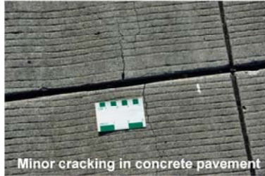
Moderate cracking in concrete pavement
