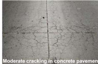
Moderate cracking in concrete pavement
