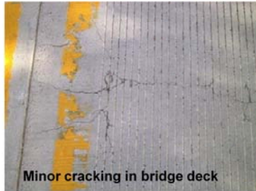
Moderate cracking in bridge deck
