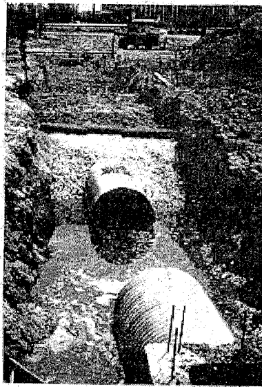
FIGURE II-3 INFILTRATION TRENCH WITH PERFORATED PIPE AND COARSE ROCK BACKFILL. NOTE GROUNDWATER LEVEL IN EXCAVATION (MIAMI AREA) (COURTESY OF DADE COUNTY DEPT. OF PUBLIC WORKS, MIAMI, FLORIDA)
