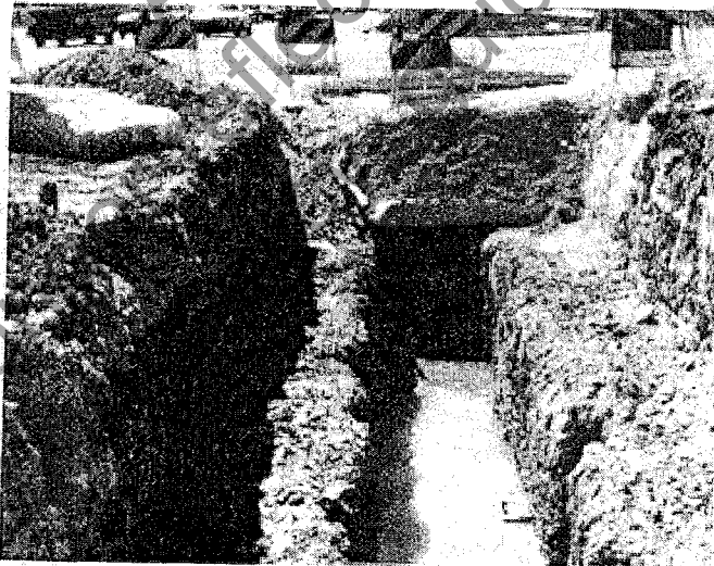
FIGURE II-2 INFILTRATION TRENCH WITH STABLE VERTICAL SIDE WALLS IN NATIVE MATERIAL WITH CONCRETE SLAB COVER (MIAMI AREA) (COURTESY OF BRISTOL, CHILDS & ASSOCIATES, CORAL GABLES, FLORIDA)
