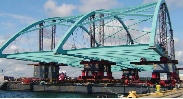
Assembled in staging area & barged to site on SPMTs Providence River Bridge, Rhode Island, 2006
