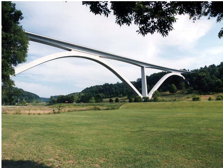
Figure 1.34 - Natchez Trace Parkway Arches, Tennessee
