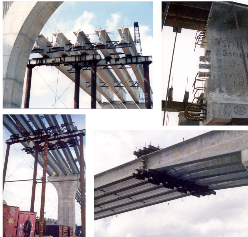
Figure 1.7 - Spliced Haunched I-Girder of Main Span Unit
