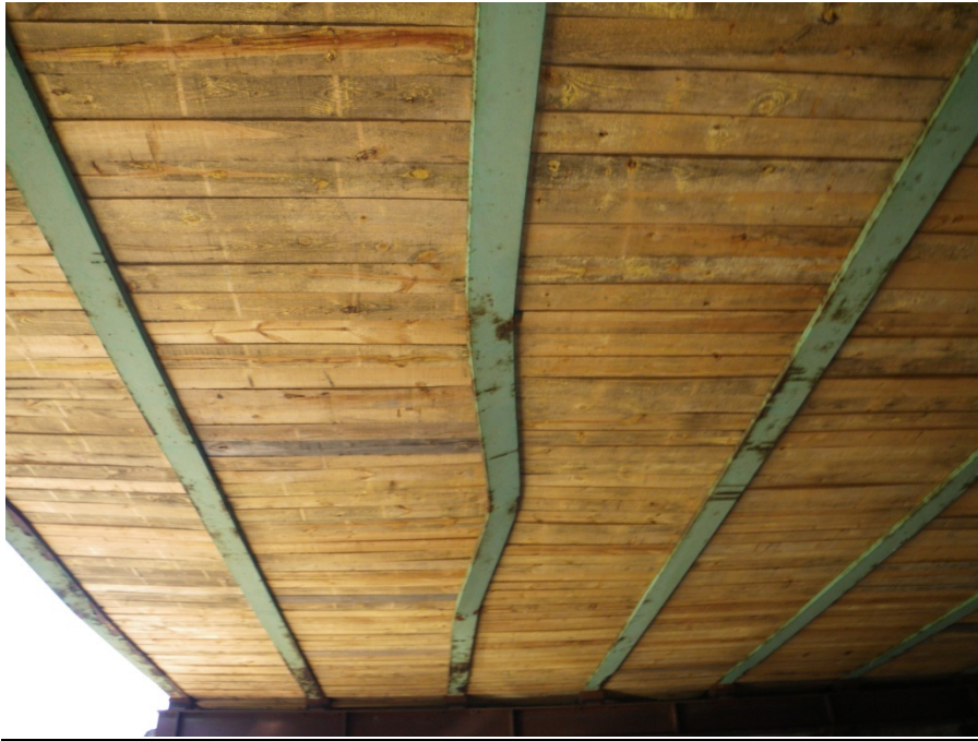
Photo A1. The underside of a steel girder bridge is shown, and one interior girder is severely distorted from collision and bent out-of-plane.
