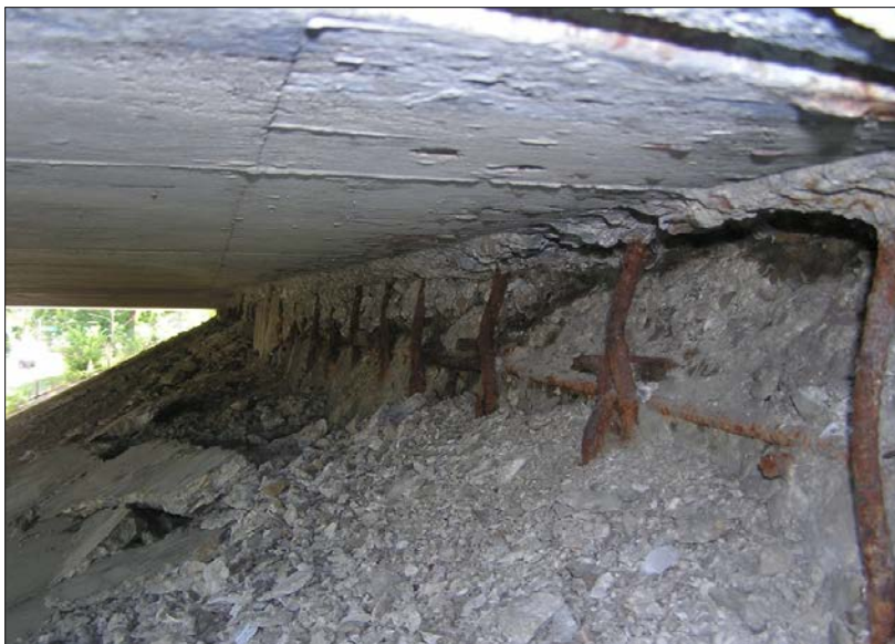
Photo 1. Shown is a deteriorated abutment that was identified as a critical finding. The reinforcing steel is corroded and deformed, and concrete is spilling down the slope wall.
