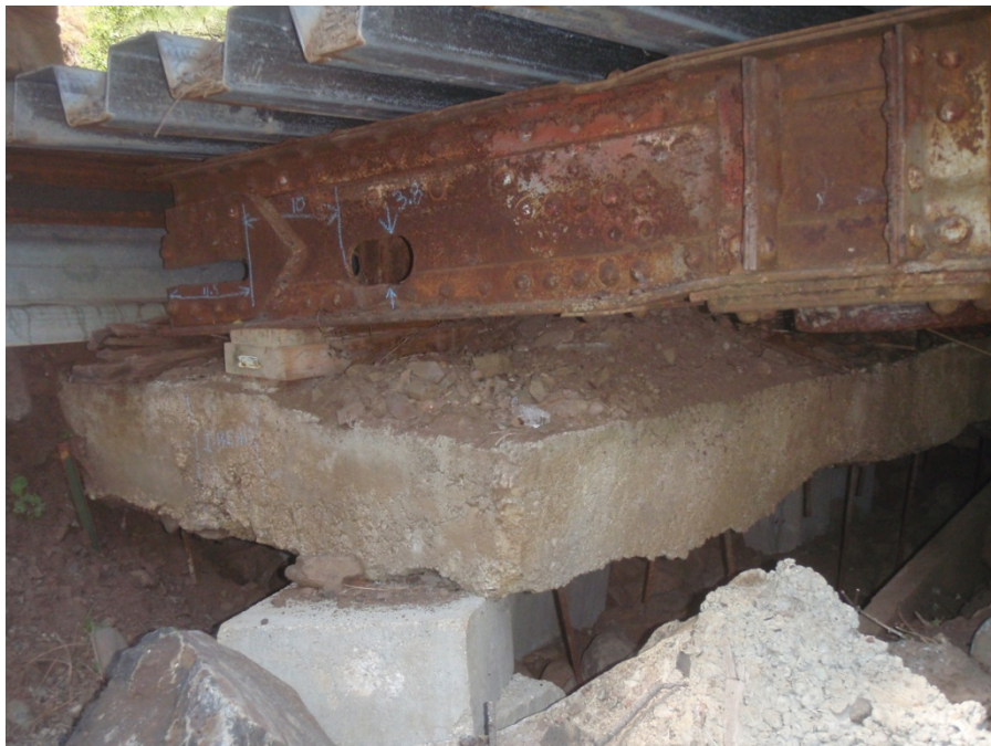
Photo A6. Shown is the underside of a bridge, and visible is a corrugated metal deck on a rail car superstructure. The end of the rail car rests on a salvaged concrete slab founded on precast concrete blocks. This repair removed an existing critical finding.
