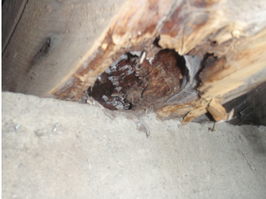
Photo A5. A close-up view of a timber stringer over a concrete abutment is shown, and the stringer is exhibiting crushing due to extensive rot and deterioration at this location.
