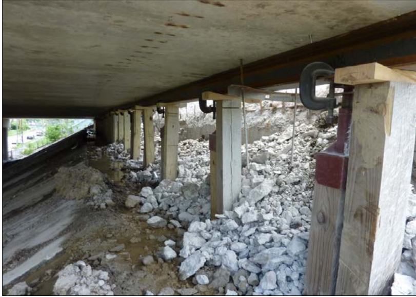
Photo 2. Temporary columns are shown that support a steel beam under the existing concrete deck, in preparation to replace the abutment that was a critical finding in Photo 1.
