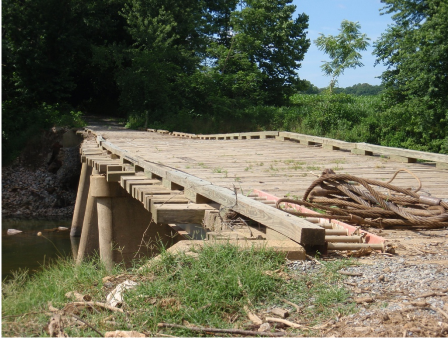
Photo A3. A timber deck on steel stringer bridge is shown. The structure has low timber guide rails, and concrete piers are tilted. The bridge is rated "3" for deck, superstructure and substructure, and the bridge is closed.
