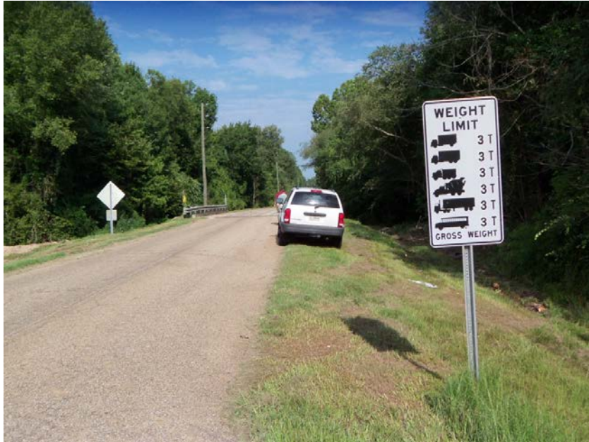
Photo 4. Shown here is a load posting sign setting the weight limit for various vehicle configurations at 3 tons. One possible outcome from a critical finding is to load post the structure.
