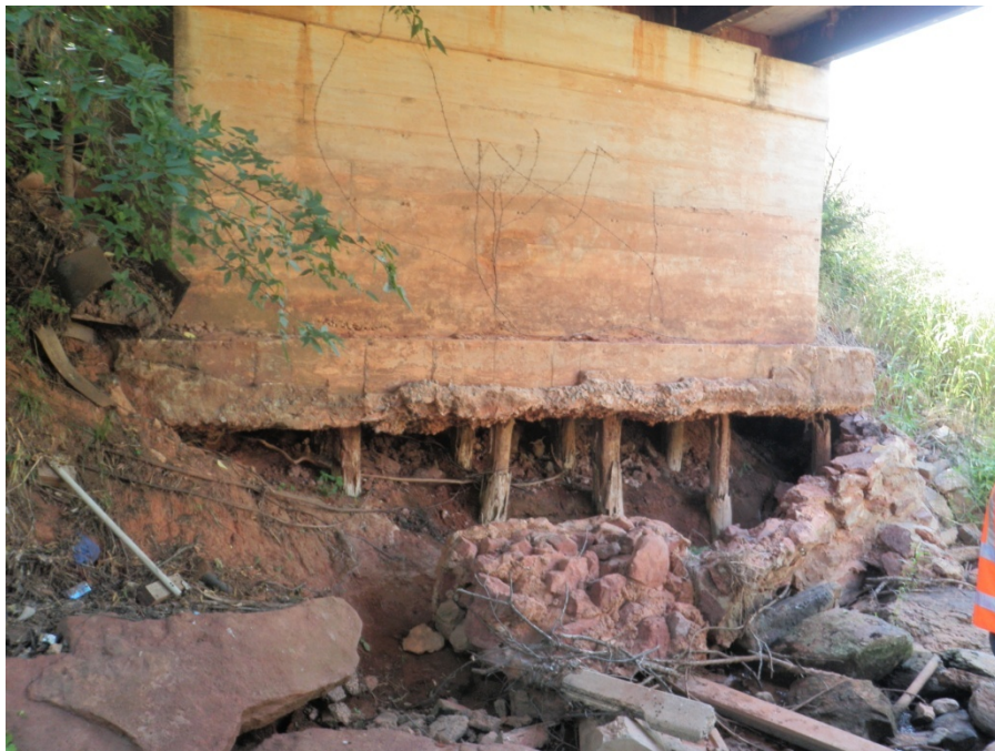
Photo A2. A concrete abutment is shown with exposed and deteriorated timber piles. There is debris in the channel and the remains of a curtain wall that once encased the pile foundation. This bridge is closed because of this critical finding.
