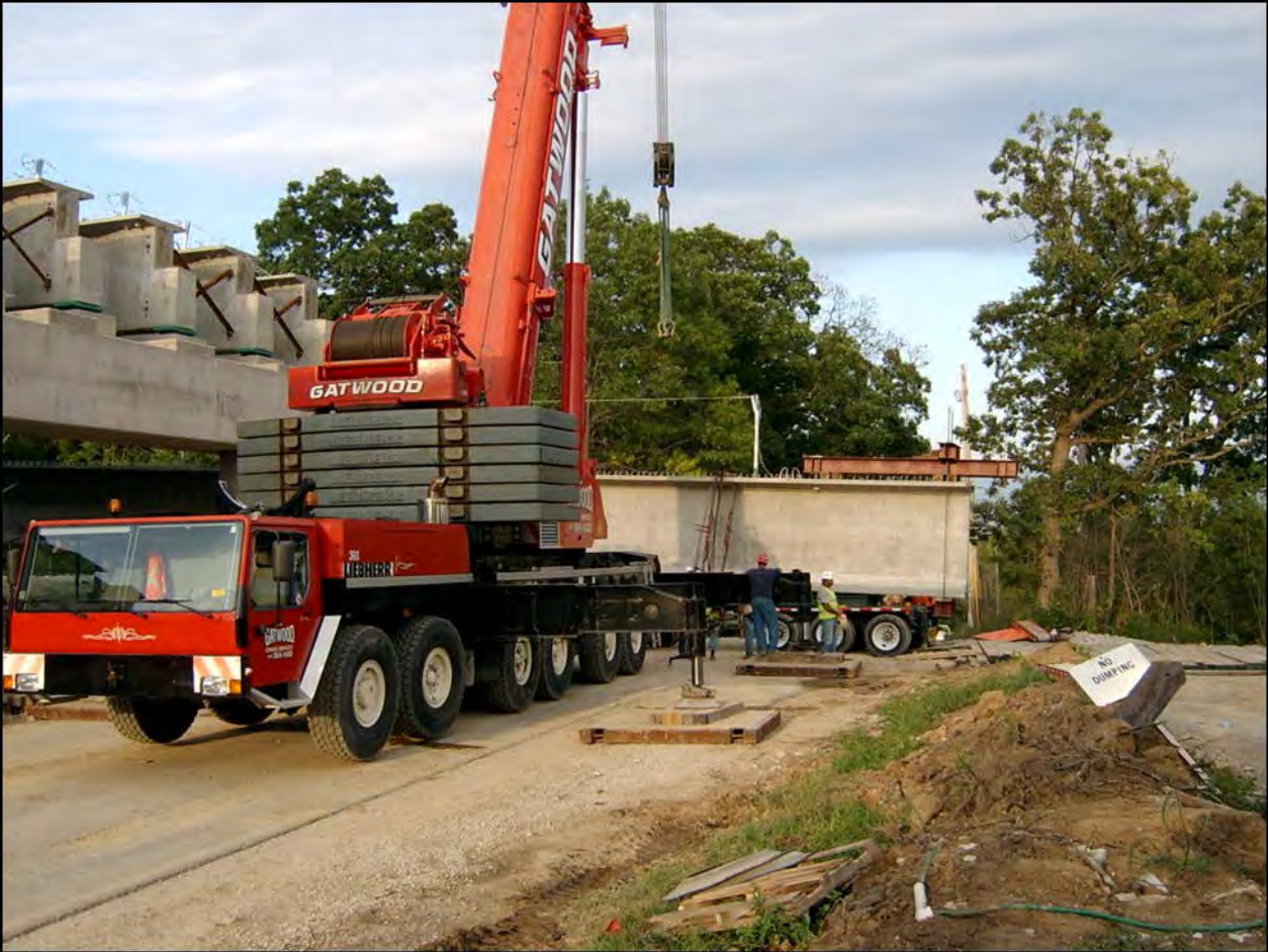
Figure 8-12 Truck Crane on Outriggers Supported on Timber Mats
