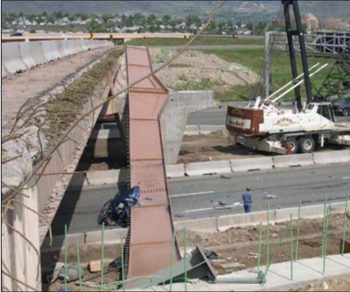
Figure 2-11 I-70 Bridge Showing Collapsed Girder
