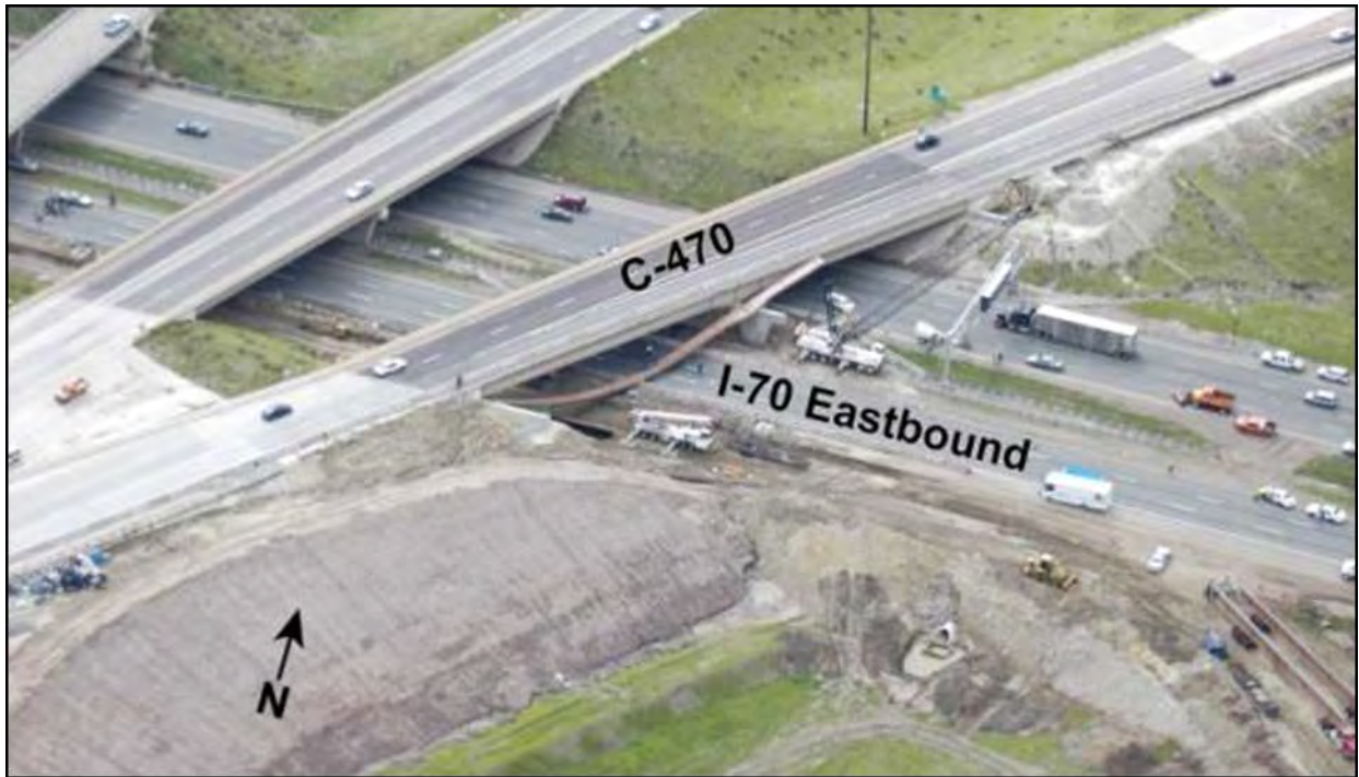
Figure 2-12 Girder Collapse - Note Girder Deflected Down Into Lane
