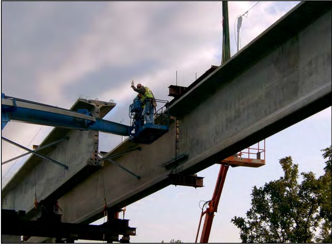
Figure 3-6 Girder Supported on Strongback (Shown on the Right)
