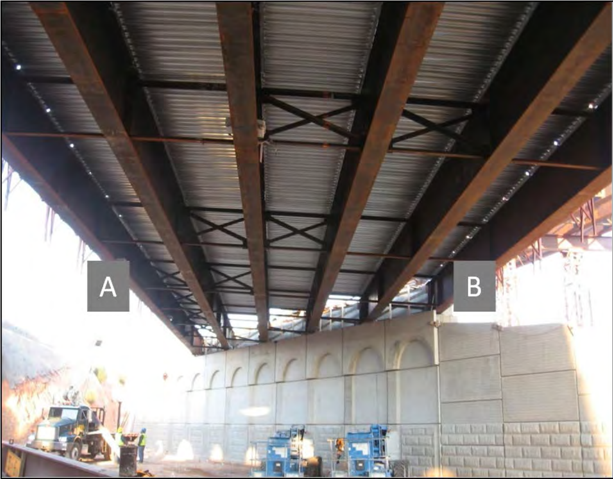
Figure 5-4 Cross-frames in Skewed Application
