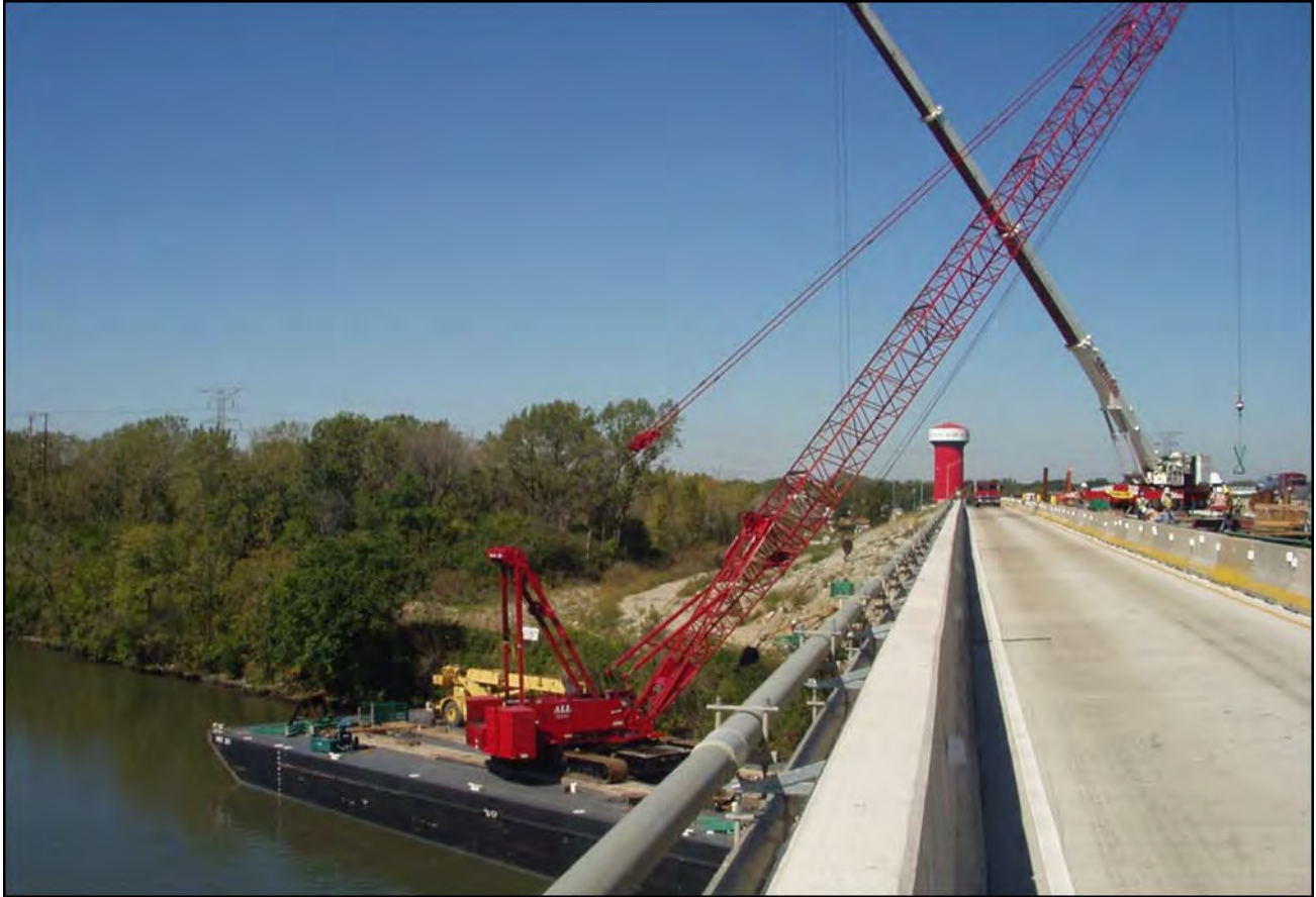
Figure 3-17 Crane Mounted on Barge
