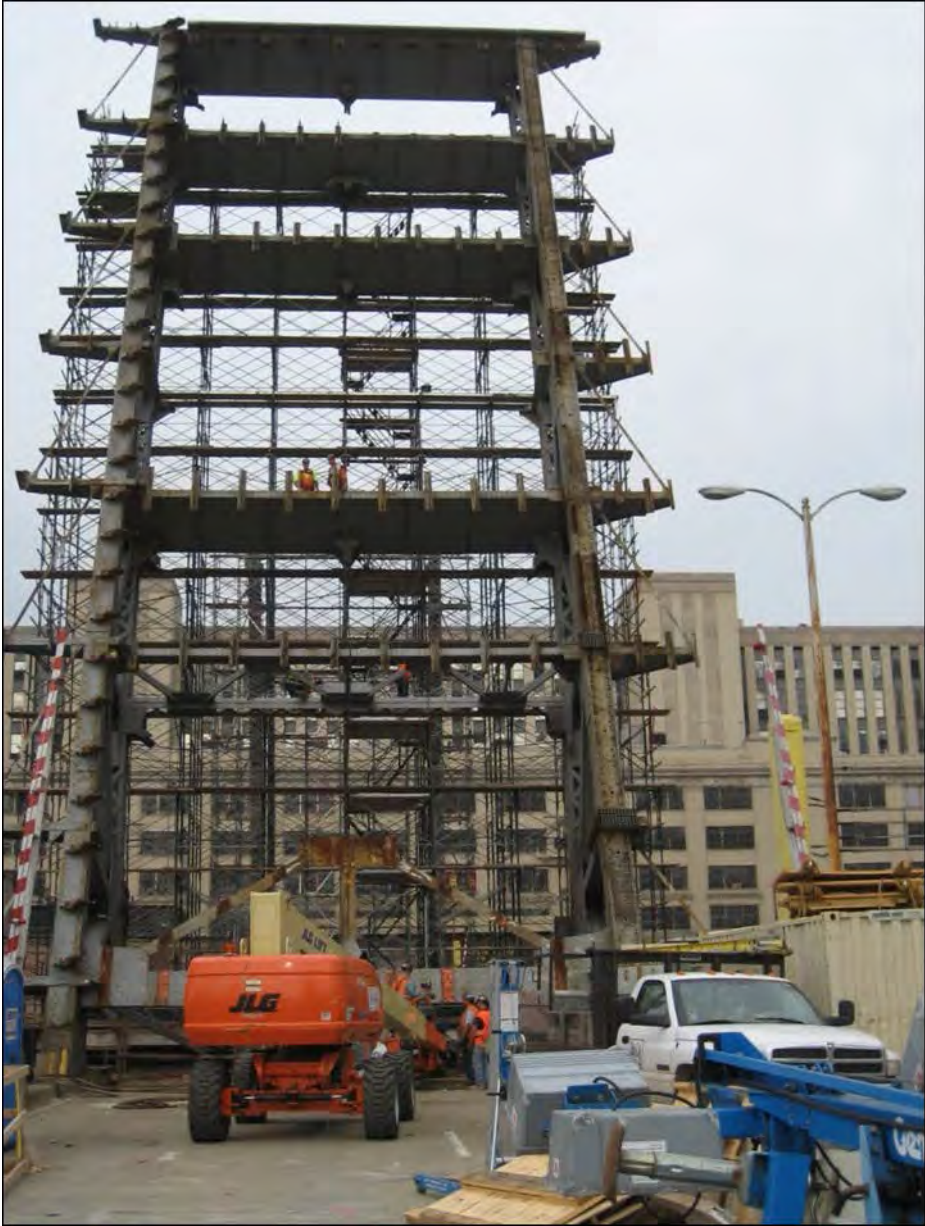
Figure 9-8 Intermediate Balancing of the Congress Avenue Bridge over the Chicago River
