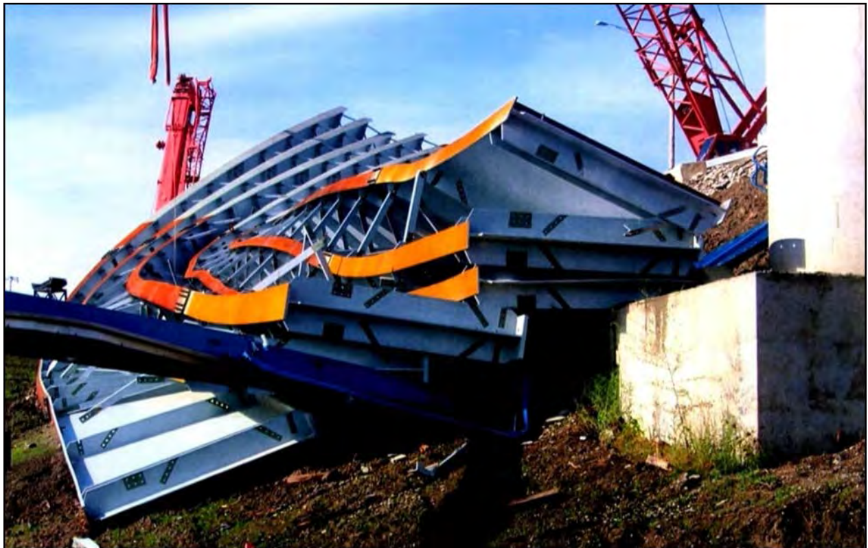
Figure 2-10 Post-Collapse Photograph - Unit 2 Looking toward Pier 6
