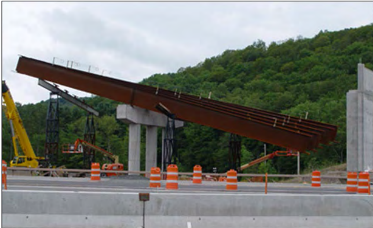
Figure 2-1 Route 17 Collapsed Shoring and Girders
