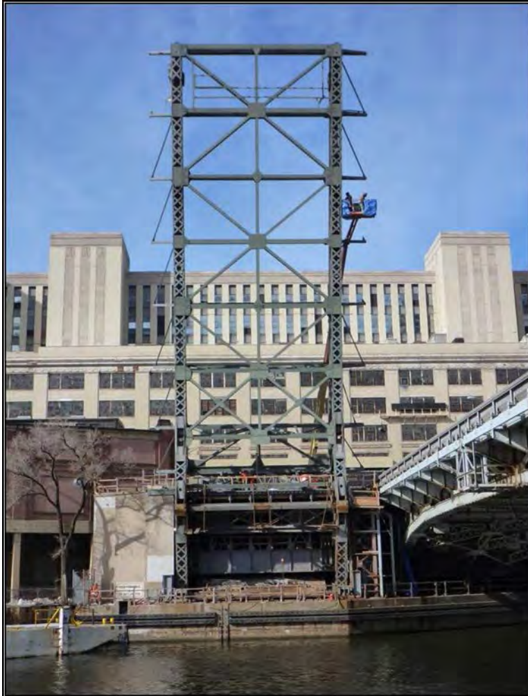
Figure 9-7 Initial Balancing of the Congress Avenue Bridge over the Chicago River
