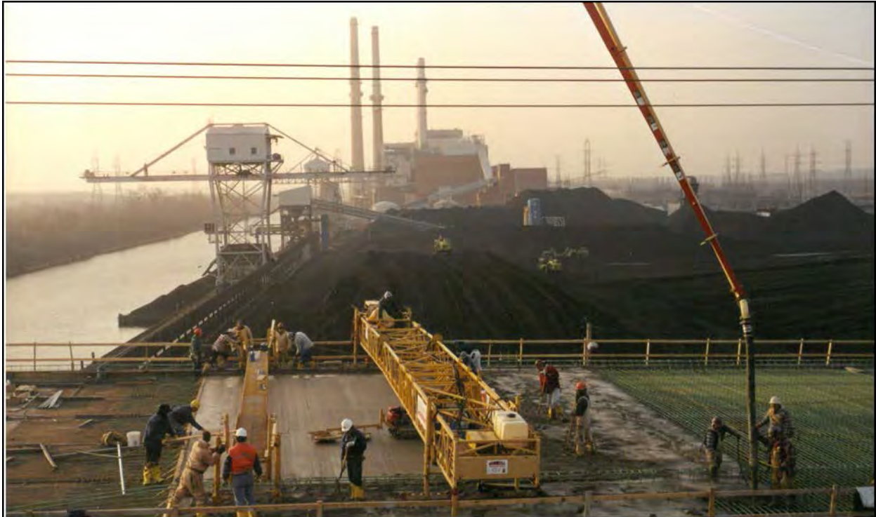
Figure 3-39 Deck Finishing Equipment for Deck Pour
