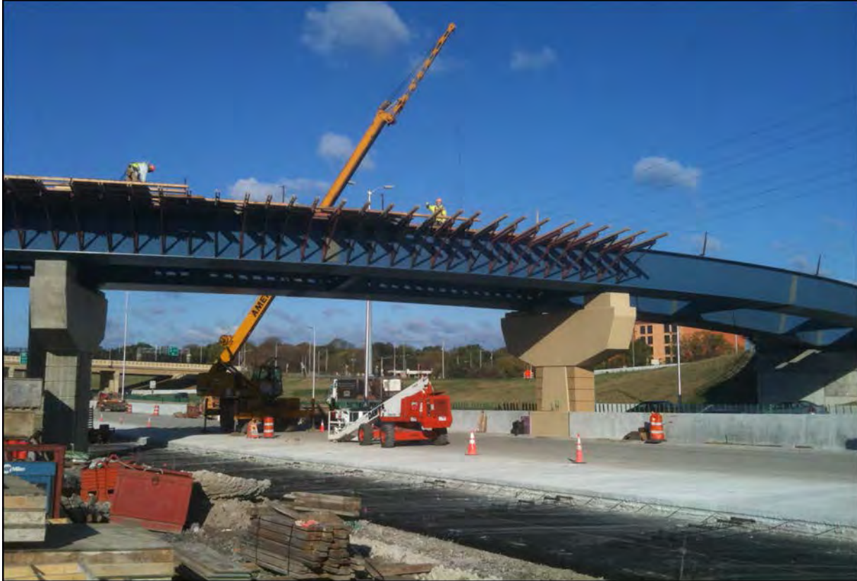
Figure 3-42 Overhang Brackets Being Set on a Tub Girder
