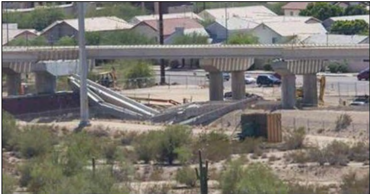
Figure 2-5 Red Mountain Freeway Showing Collapsed Concrete Girders on Ground
