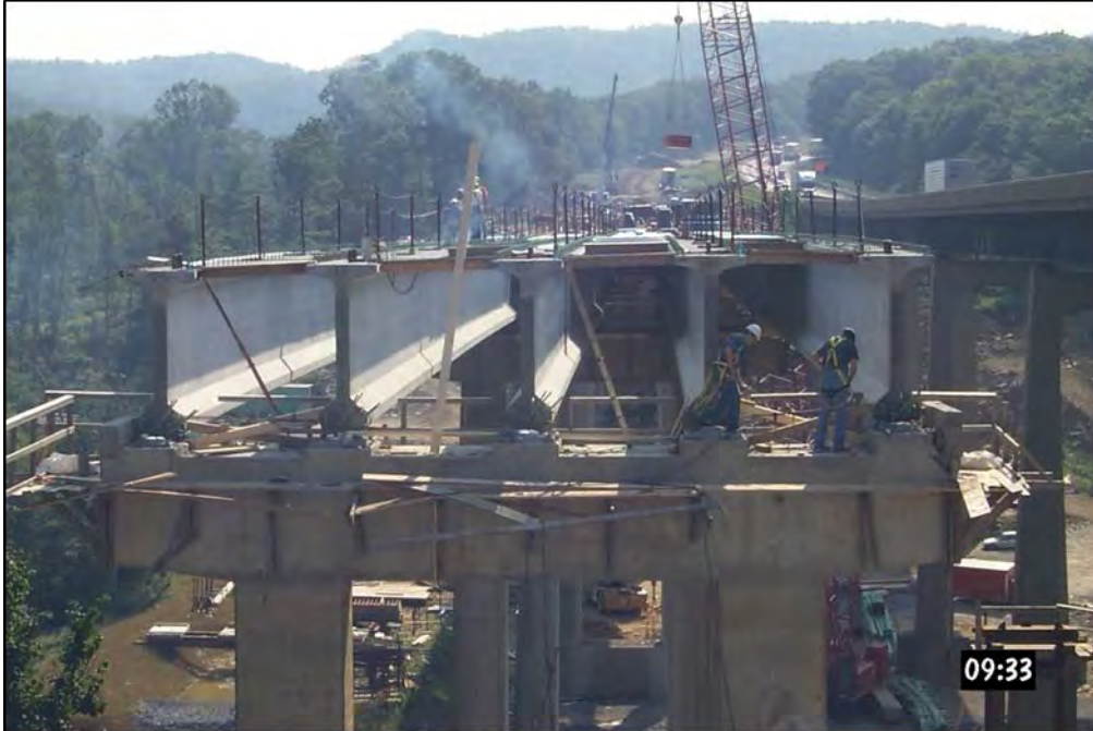
Figure 2-21 End view of I-80 Bridge under Construction Prior to the Collapse
