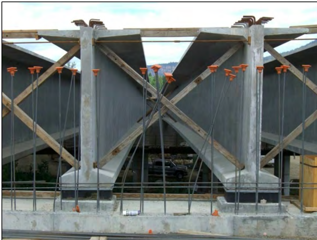
Figure 3-32 Timber X-Bracing for Concrete I-girders
