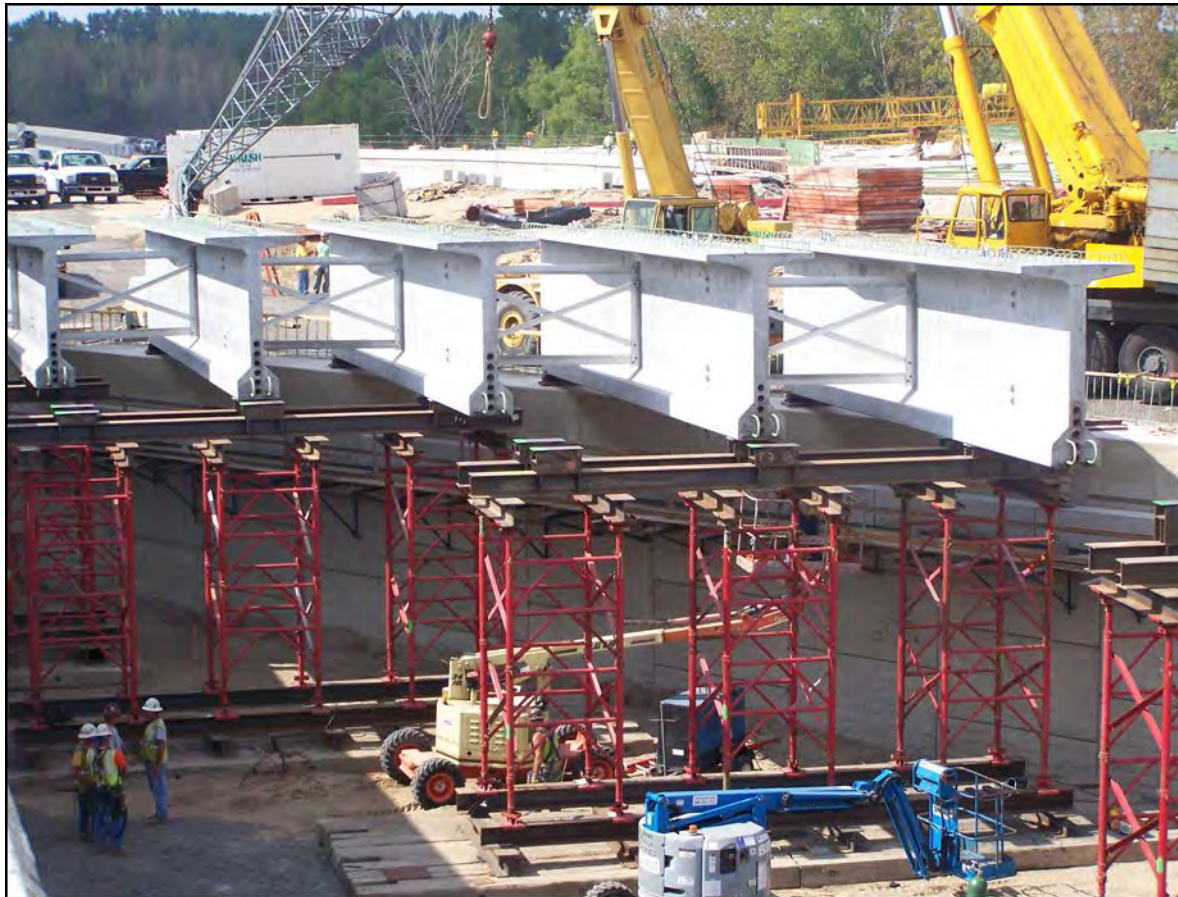
Figure 3-38 Shoring Towers Supported on Timber Mats
