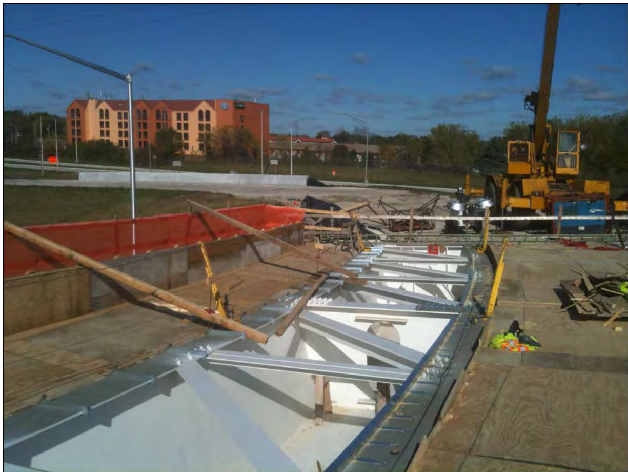
Figure 3-23 Box Girder Top Lateral Bracing and Diaphragms
