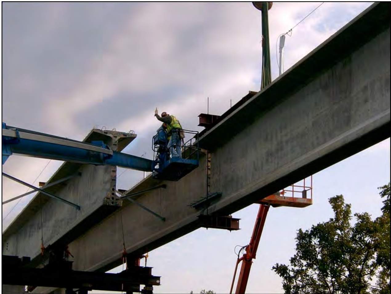
Figure 8-15 Precast Concrete Girder Supported on Strongback
