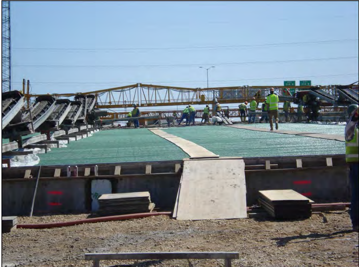
Figure 7-4 Concrete-placing and Finishing Equipment on Bridge Deck
