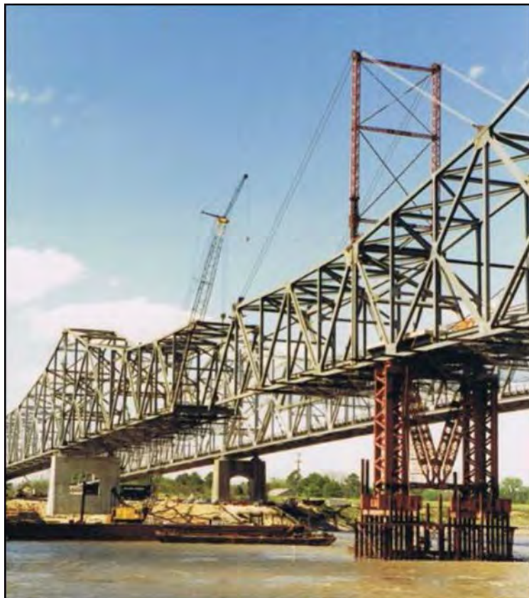
Figure 9-5 Temporary Kingpost Supporting Cantilever Construction of Bridge Truss Over the Mississippi River
