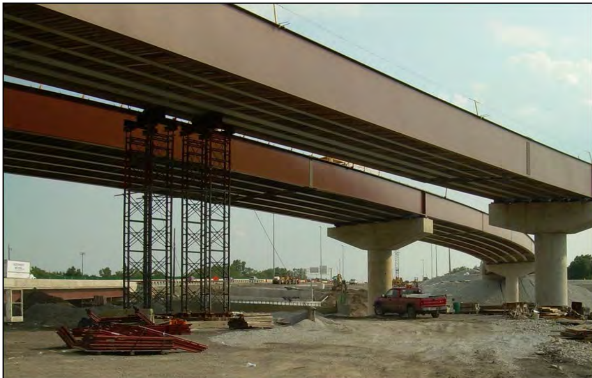
Figure 3-36 Shoring Towers Supporting Girders during Erection
