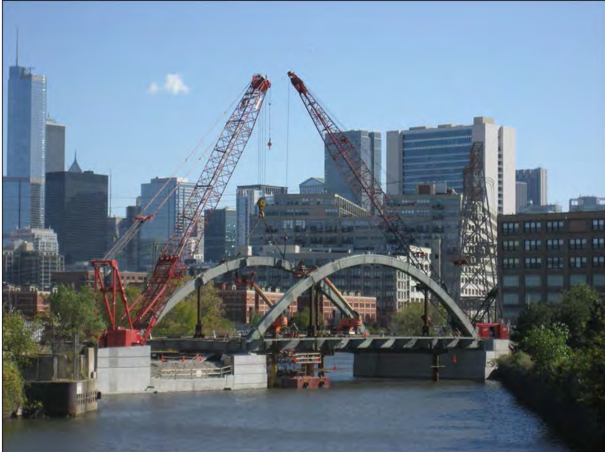
Figure 9-3 Erection of Tied Arch Bridge Using Falsework
