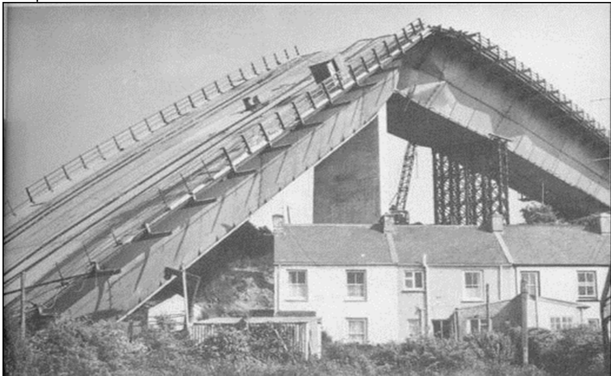
Figure 2-22 Cleddau Bridge Buckled over Pier
