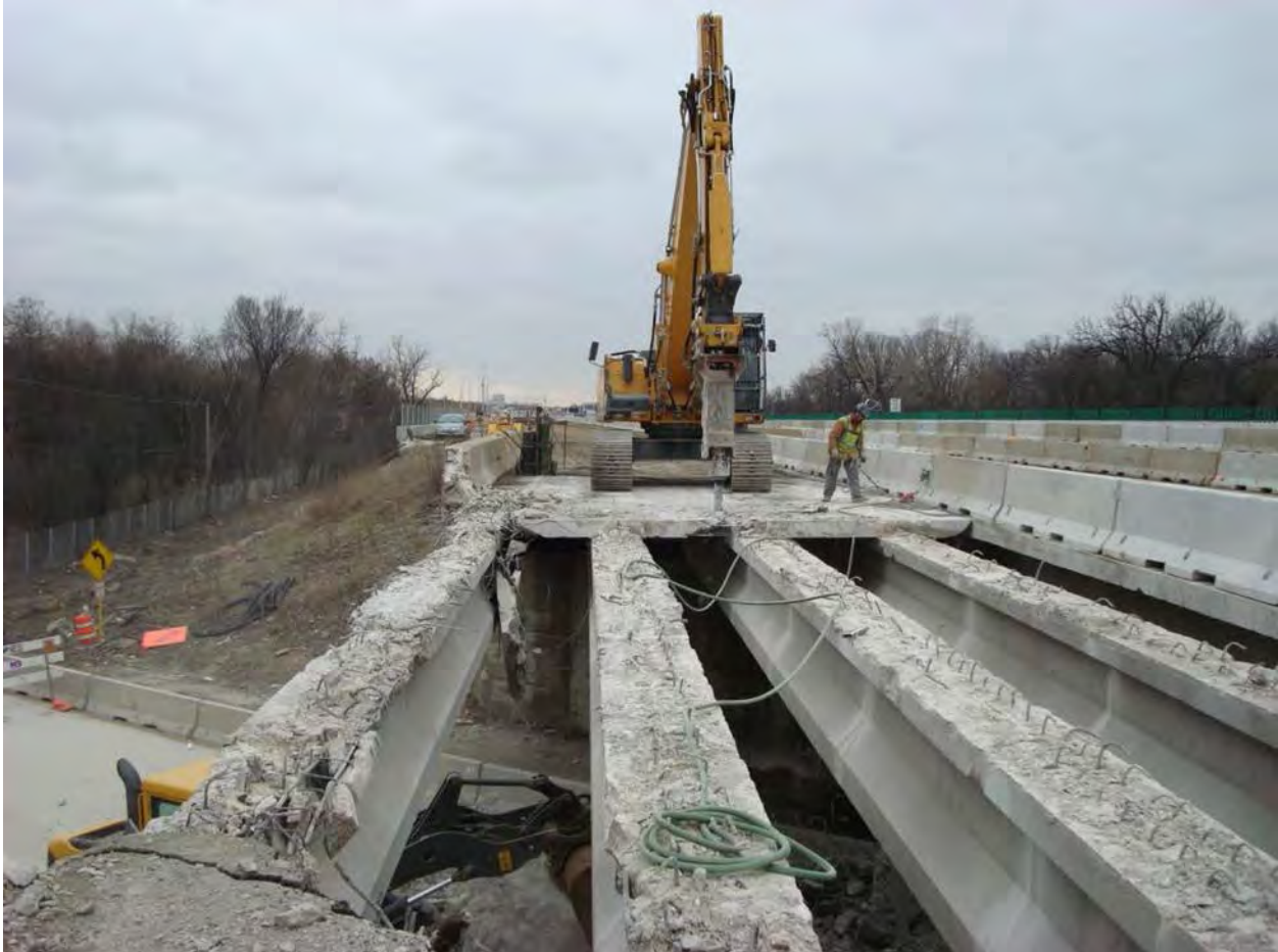
Figure 3-44 Bridge Deck Demolition Removing Deck in Sections
