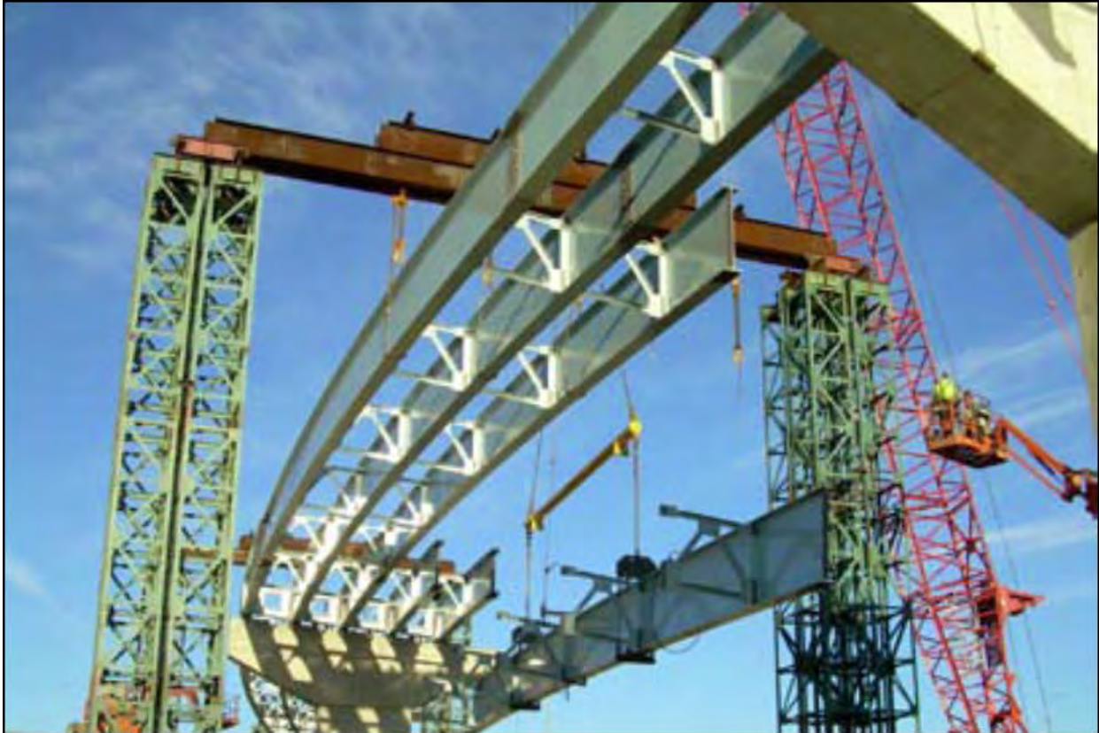
Figure 3-4 Curved Girder Being Erected with Cross-Frames Attached
