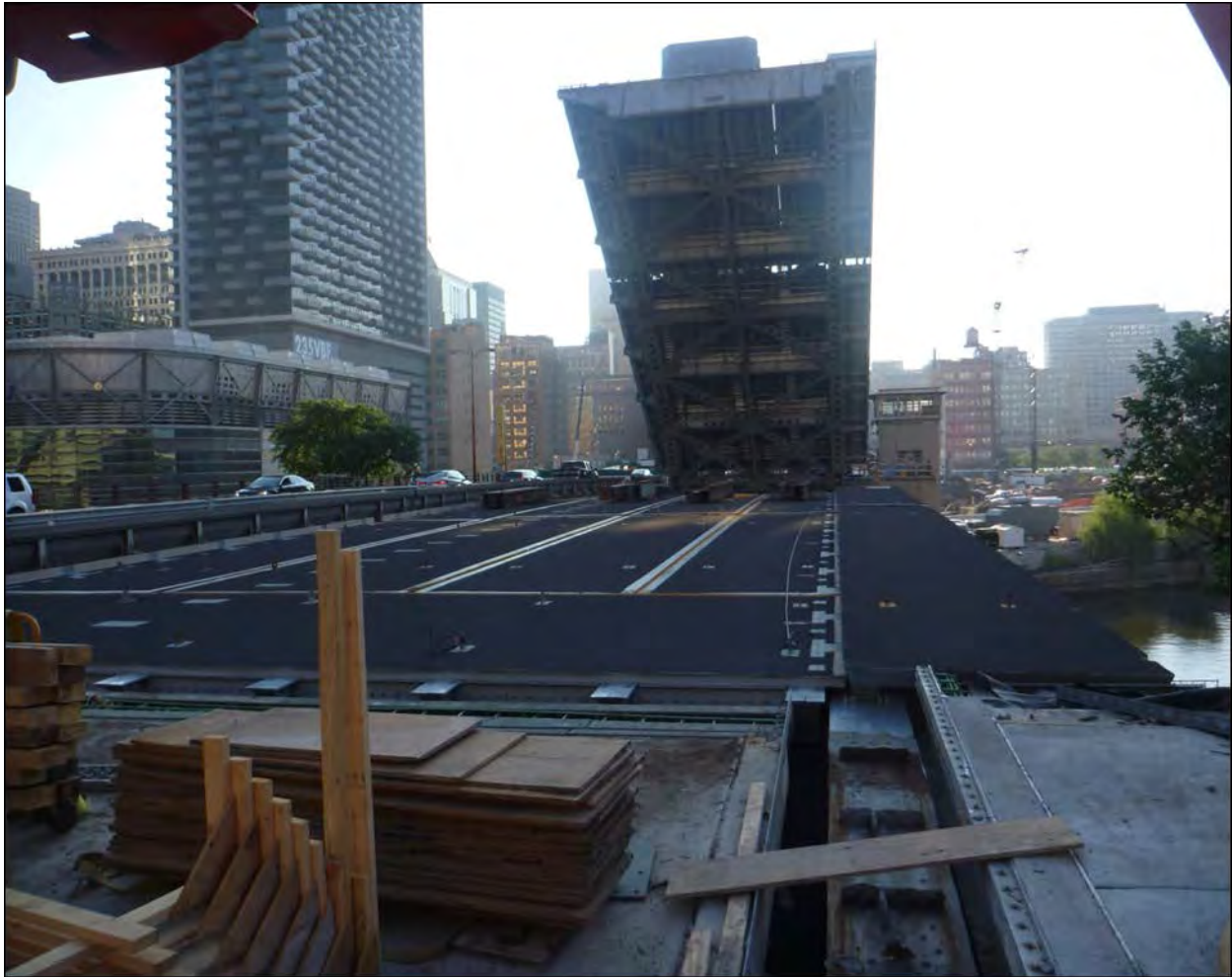
Figure 9-9 Late Stage Balancing of Congress Ave Bridge over the Chicago River
