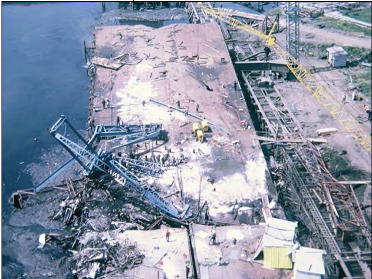
Figure 2-23 West Gate Bridge after Collapse
