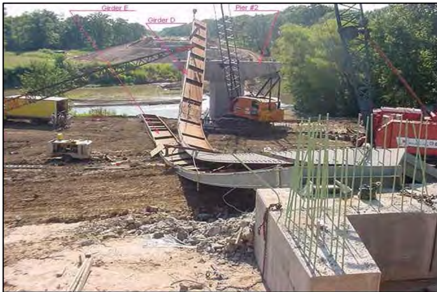
Figure 1-1 Collapse of Steel Girder Bridge during Construction
