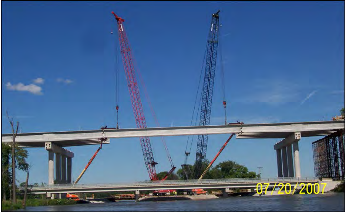
Figure 3-5 Setting Drop-in Span with Strongbacks Attached
