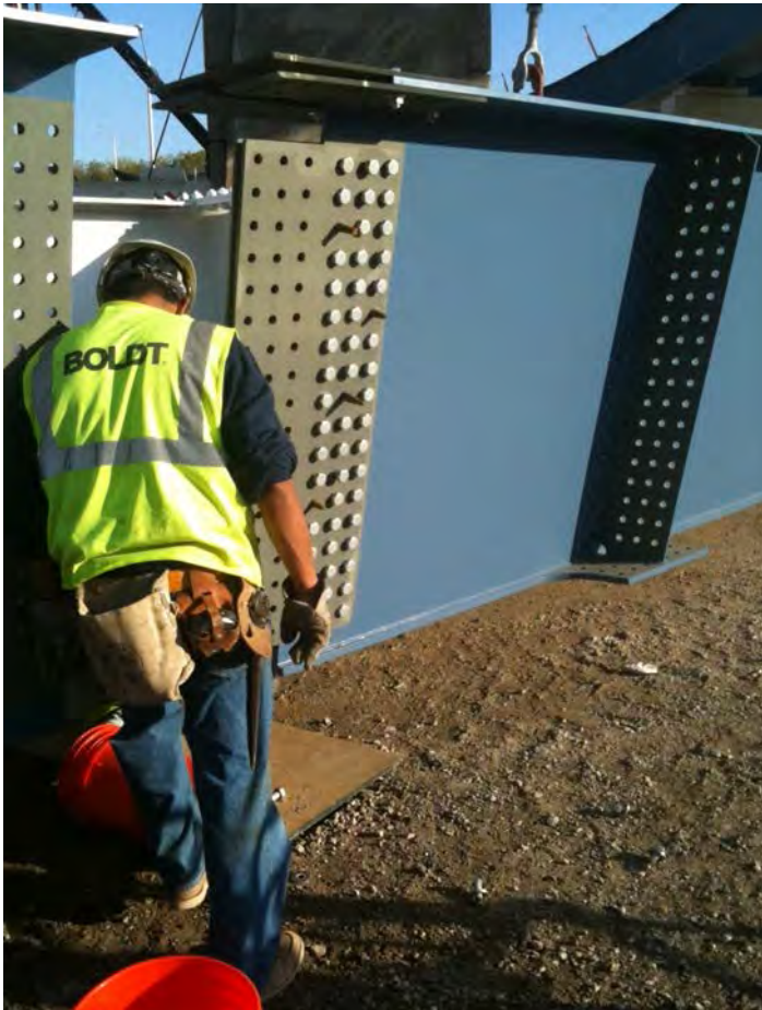
Figure 3-3 Splicing Girder Segments at Grade Prior to Lifting
