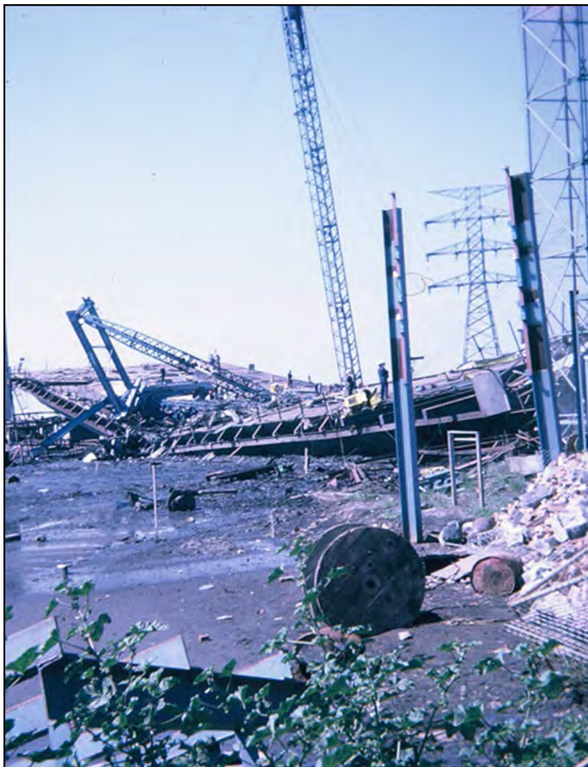
Figure 2-24 West Gate Bridge Construction Site after Collapse
