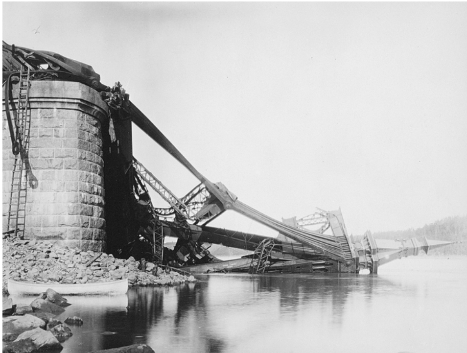
Figure 2-17 Quebec Bridge after Collapse (Modjeski et.al, 1919 – used by permission of Library and Archives of Canada)
