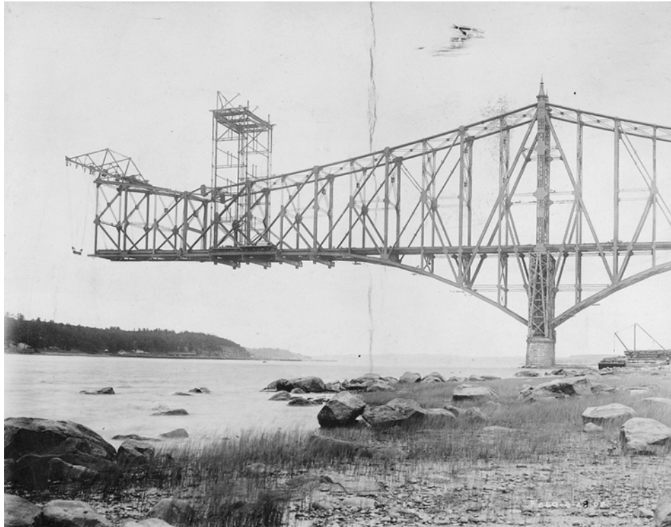
Figure 2-16 Quebec Bridge under Construction Shortly before Collapse (Modjeski et.al, 1919 – used by permission of Library and Archives of Canada)
