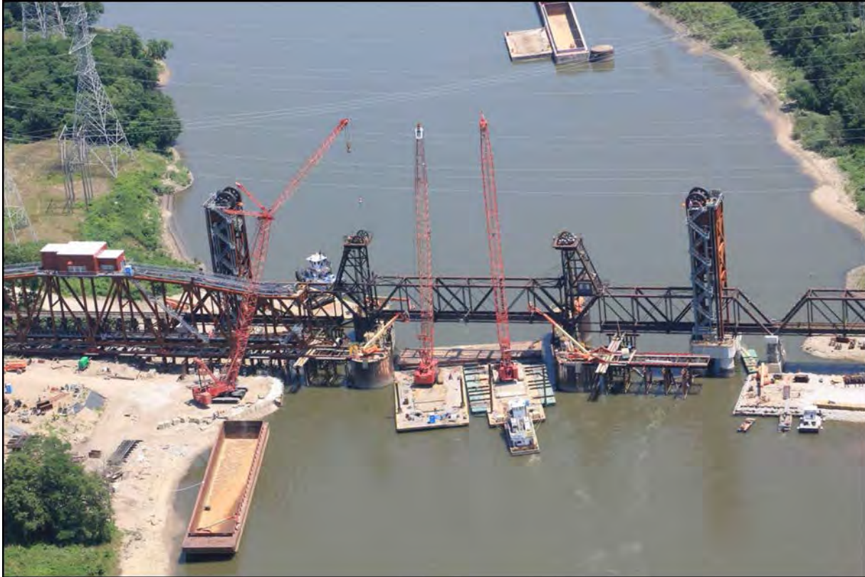
Figure 9-6 New Truss on Temporary Trestle for Slide-In
