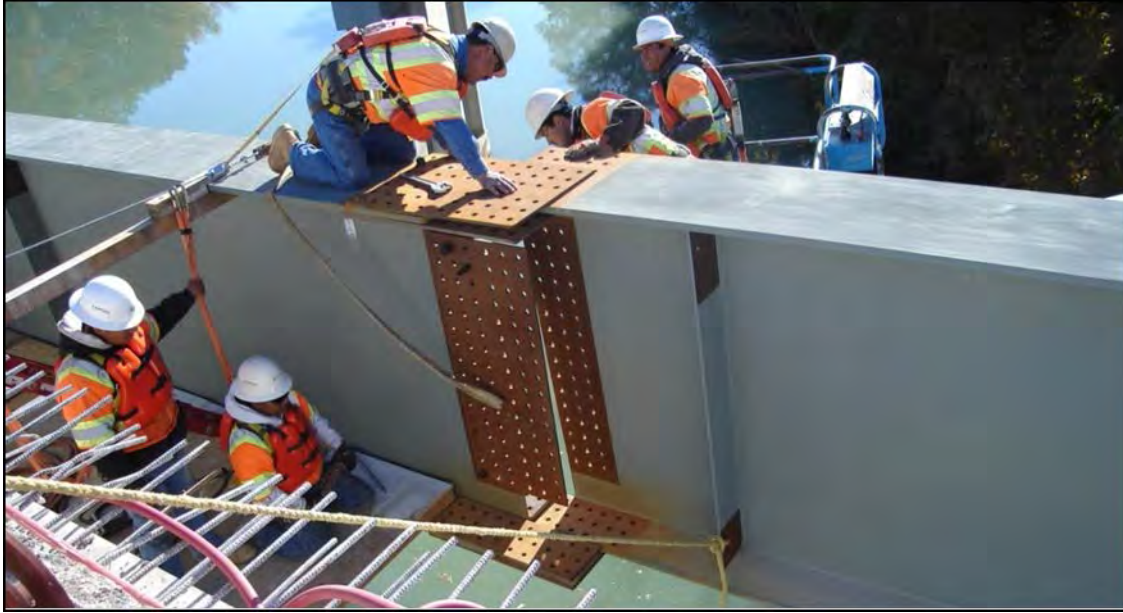
Figure 6-14 Bolted Air Space [Stith et al. 2010]
