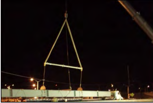
Figure 3-13 Spreader Beam
