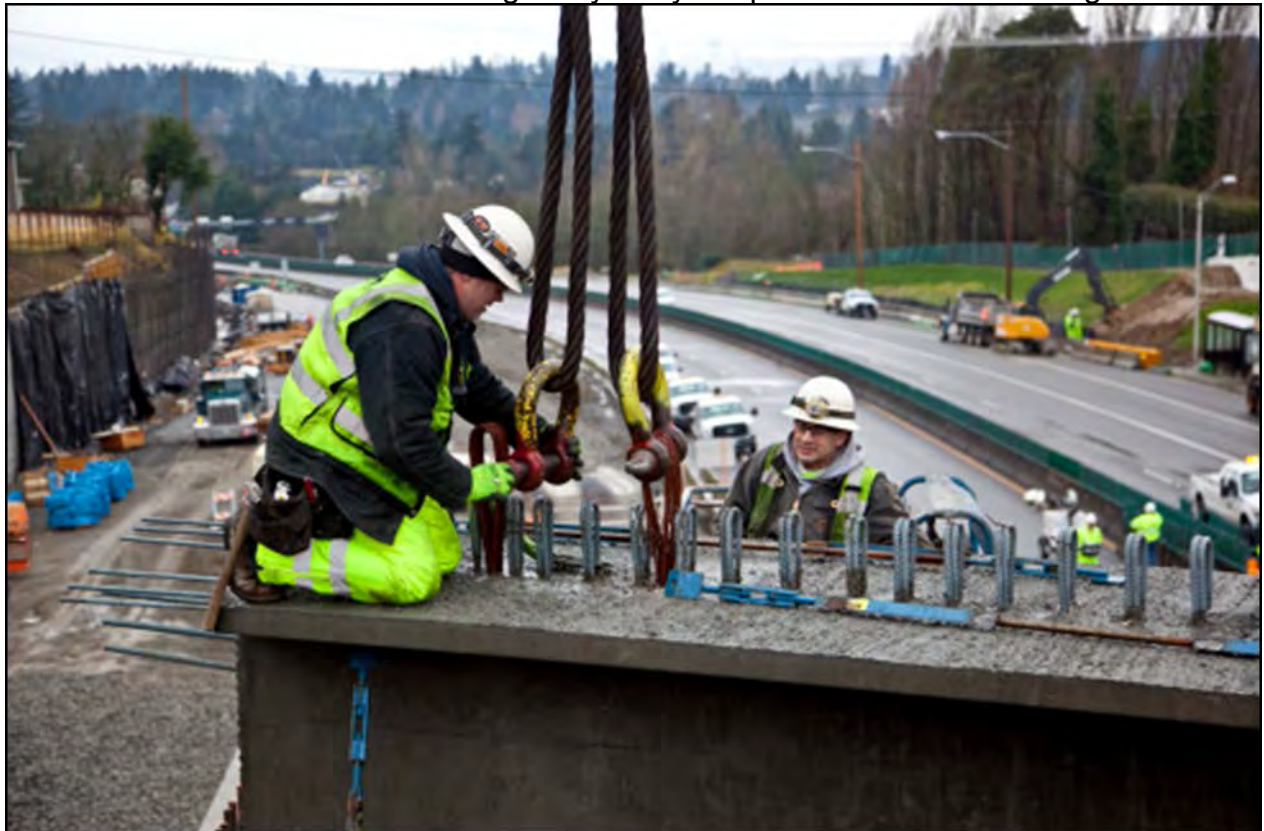
Figure 3-10 Crane Rigged to Concrete Girder at Lifting Loops
