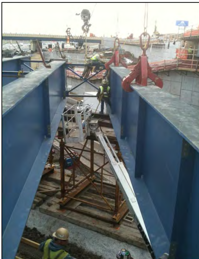
Figure 3-9 Beam Clamps on Steel Girder
