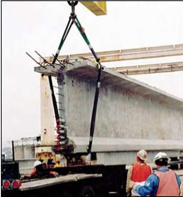
Figure 3-11 Basket Hitch Rigging
