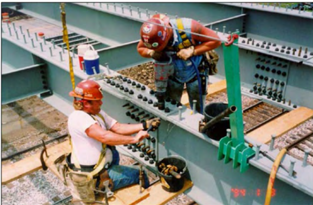
Figure 3-15 Girder Splice Bolts Being Installed and Drift Pins in Place
