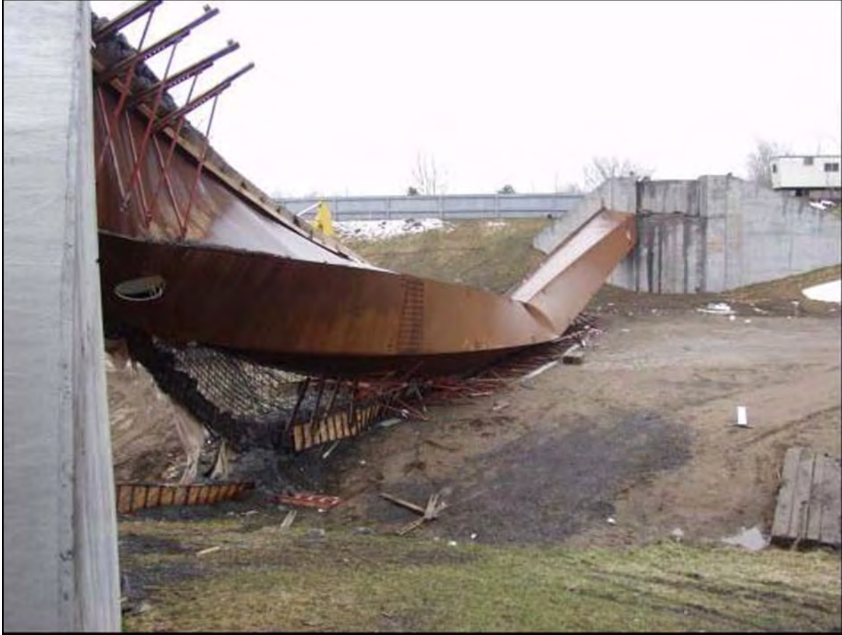
Figure 2-4 Marcy Bridge after Collapse
