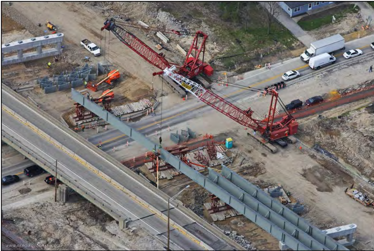
Figure 3-20 Multiple Cranes Lifting Girder – Aerial View
