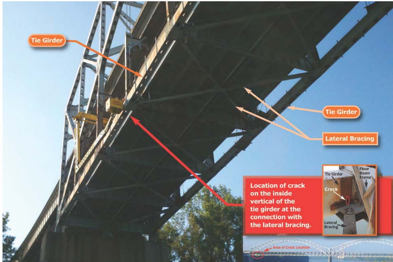
Figure 1. Location of crack initially responsible for closing the Sherman–Minton Bridge.
