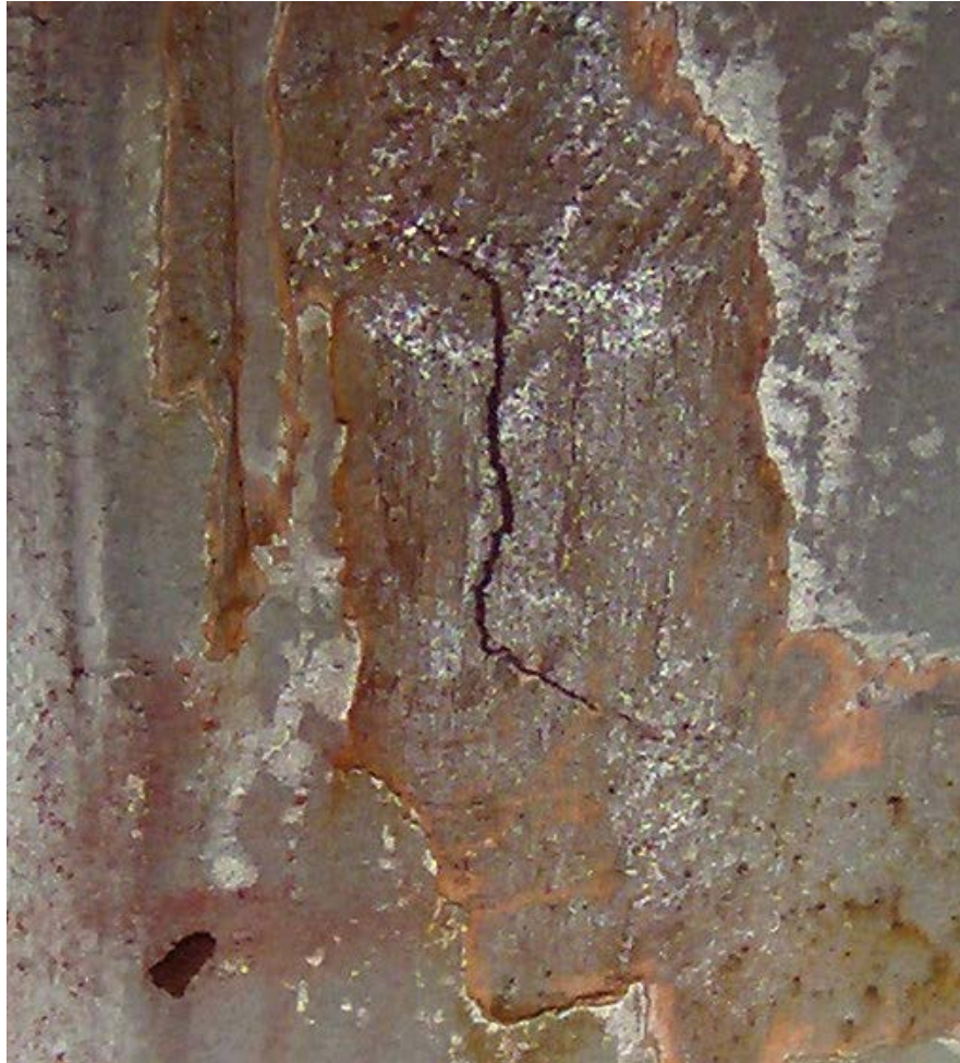
Figure 2. A crack measuring approximately 2 1/8 inches long by 1 1/4 inches deep in the side plate of the south tie of span 2 of the Sherman-Minton Bridge.
