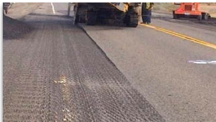
In some spots there was near zero depth to mill and maintain the sub structure for the whitetopping.
