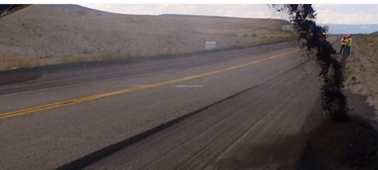
Milled Segment of I-70 Reveals Asphalt Depth Variance.
