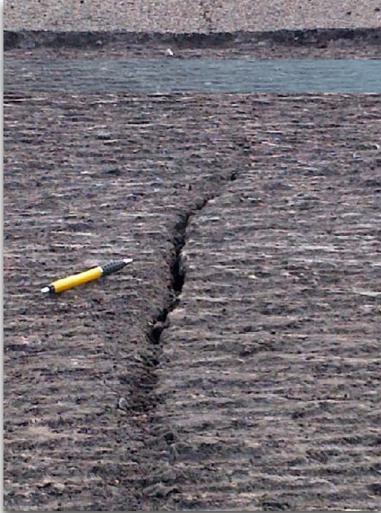
Deeply cracked asphalt on a milled section of I-70 illustrates the poor condition of some of the existing pavement.
