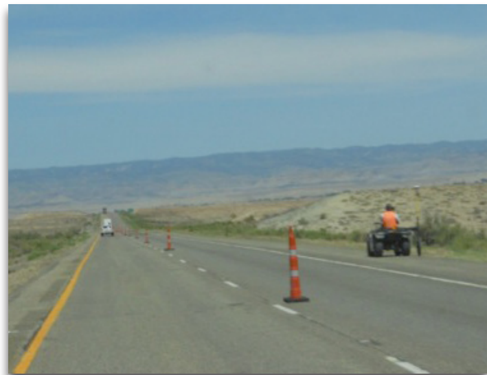
The winning contractor conducted five passes at 25 ft intervals on both eastbound and westbound lanes for a GPS survey.
