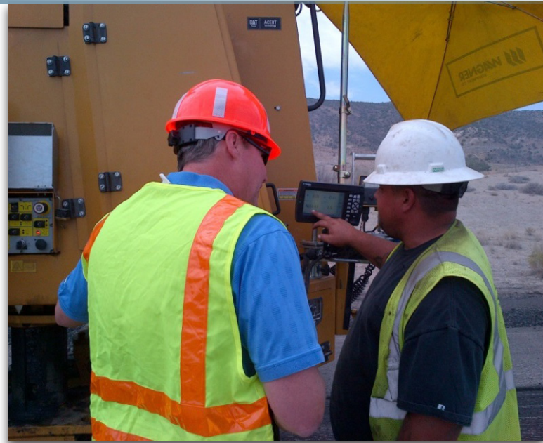
The machine operator reads the screen, which tells him where there are deviations from the pre-set model.
