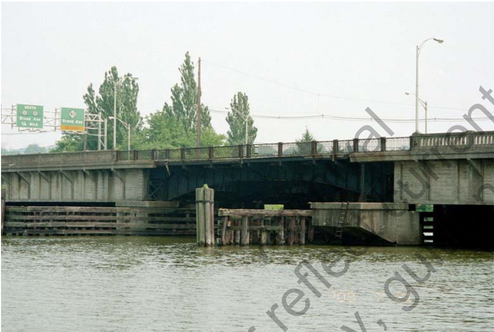
Route 46 bridge spanning Overpeck Creek
